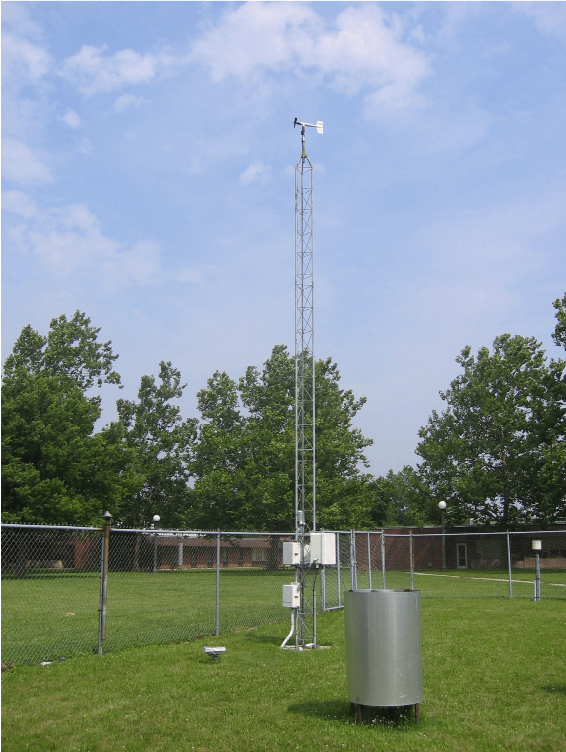
Figure 2-36 Photo of Meteorological Tower at U. of I.
