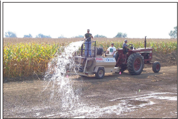
Applying PAM solution with a hydroseeder to a newly constructed grass waterway channel.
