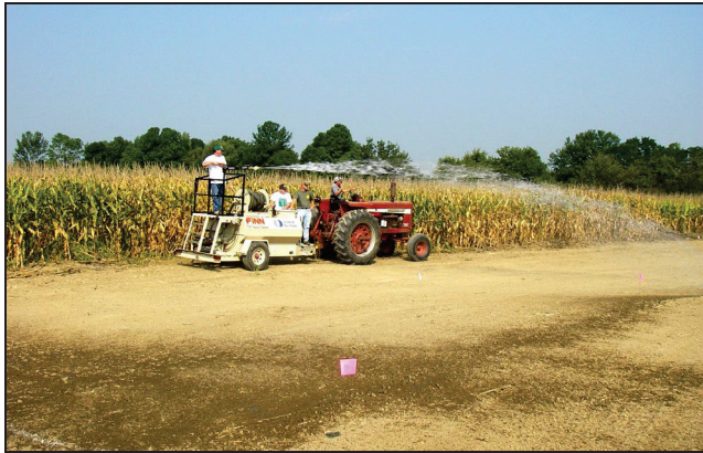
Applying PAM solution with a hydroseeder to a newly constructed grass waterway channel.
