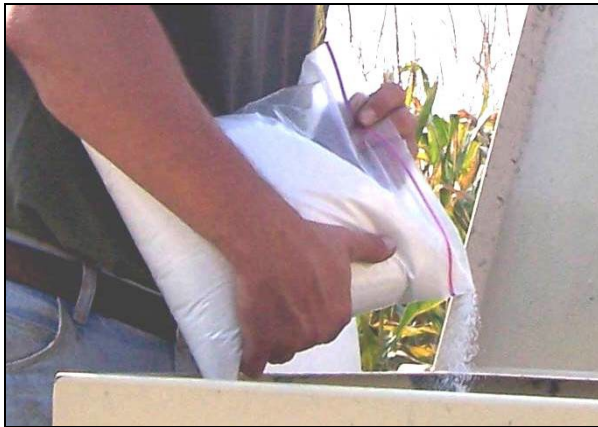
Adding PAM dry powder to a hydroseeder tank.
