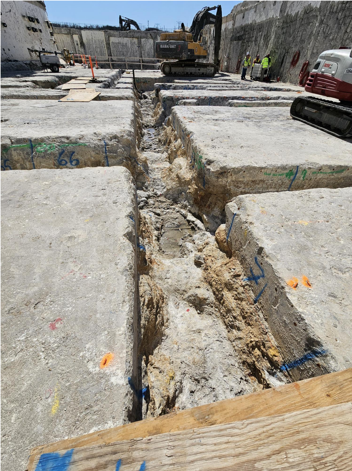
Figure 1 – Wetted areas of Trench 16 after infiltration event
