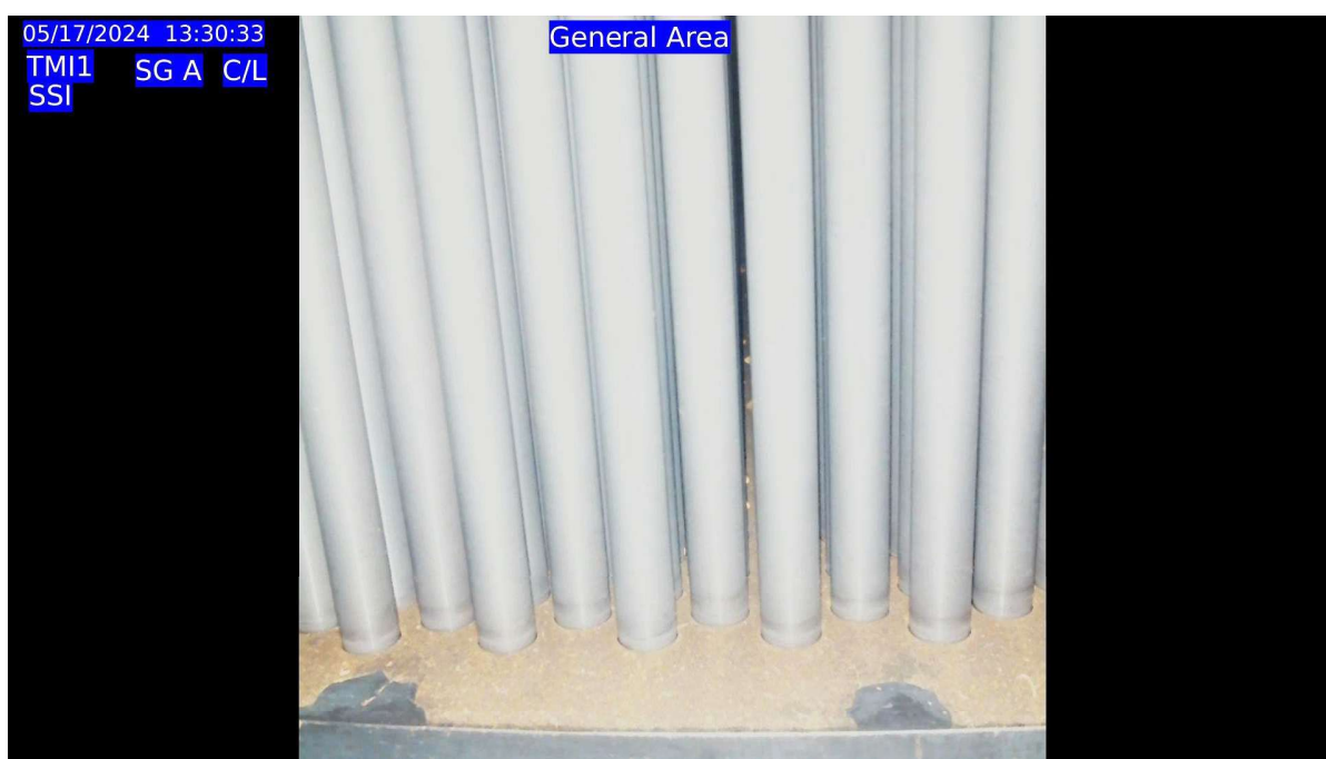
Figure 6-1: TMI-1 SG A Secondary Side As-Found View
