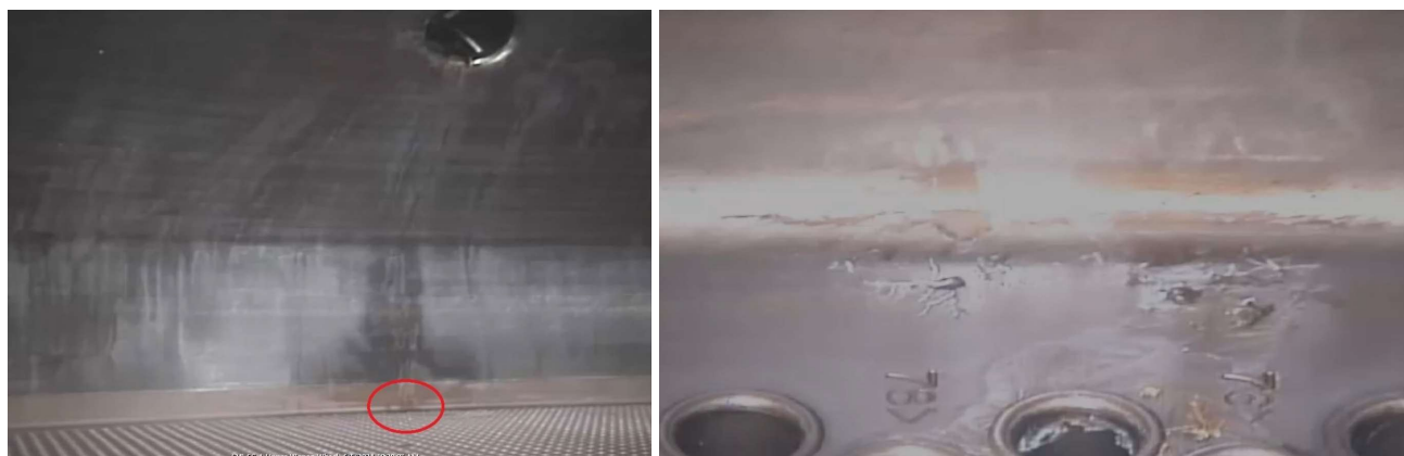
Figure 4-27: CR 2024-1448: Suspect Foreign Material in SG A Upper Head
