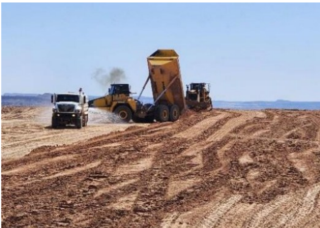
Photo 14. RRM Placement and Dust Control. April 2025
