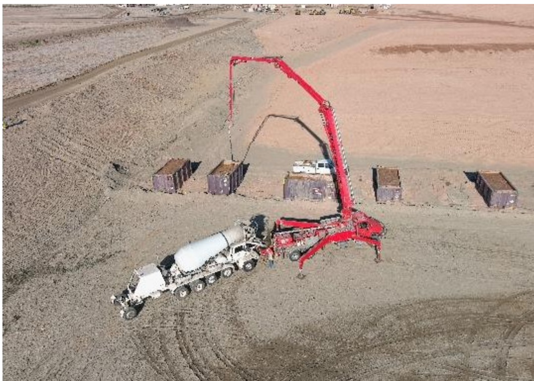
Photo 17. One Trip Containers Receiving Flowable Fill to Minimize Voids. June 2025
