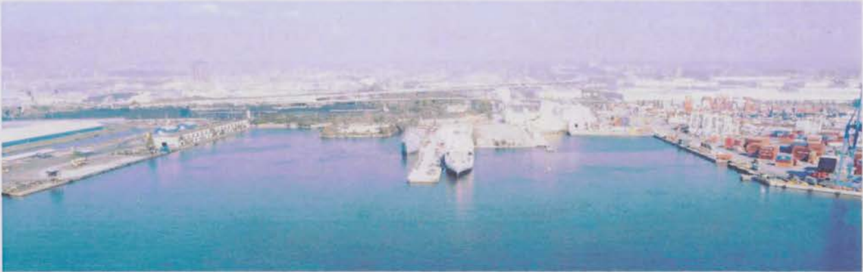
Figure 1-11 NSS at Pier 13, September 2023, looking northward
