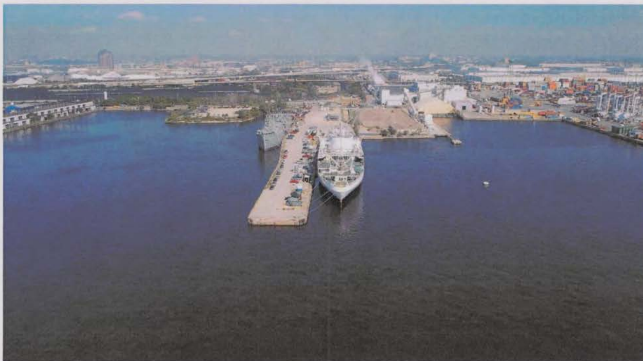
Figure 1-10 NSS at Pier 13, September 2023, looking northward
