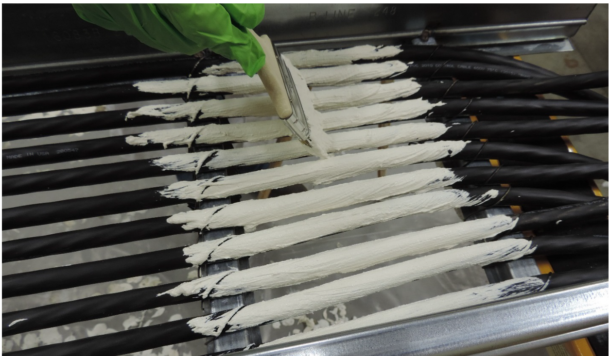
Figure 6-5. Application of FS15 cable coating by paintbrush.
