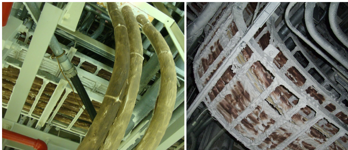
Figure 6-1 Cable coatings showing change from their original white color
