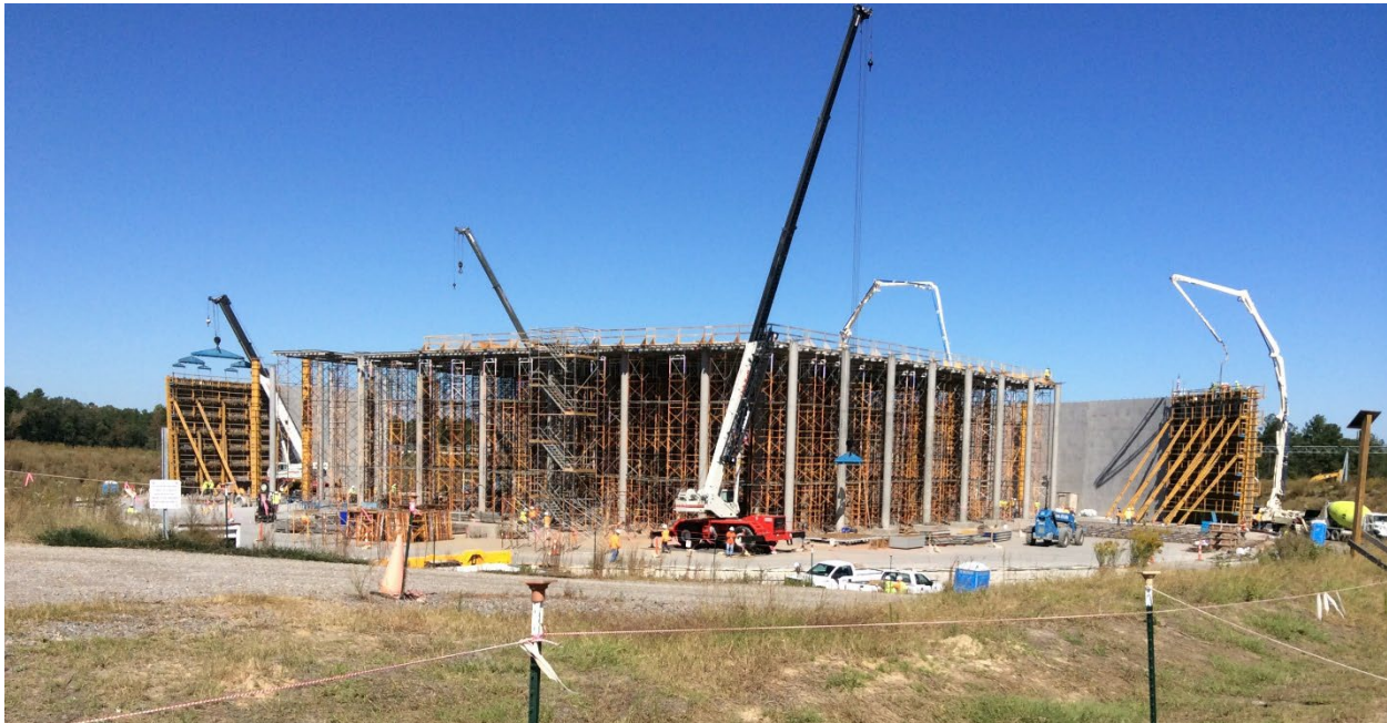
Figure 2.2-1: Construction of SDU 6, October 2014
