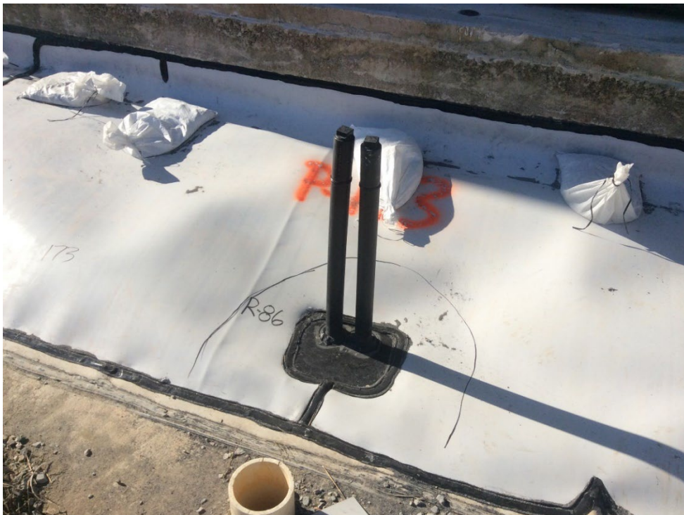
Figure 2.3-9: Installation of HDPE Over the Mud Mats at East Sump
