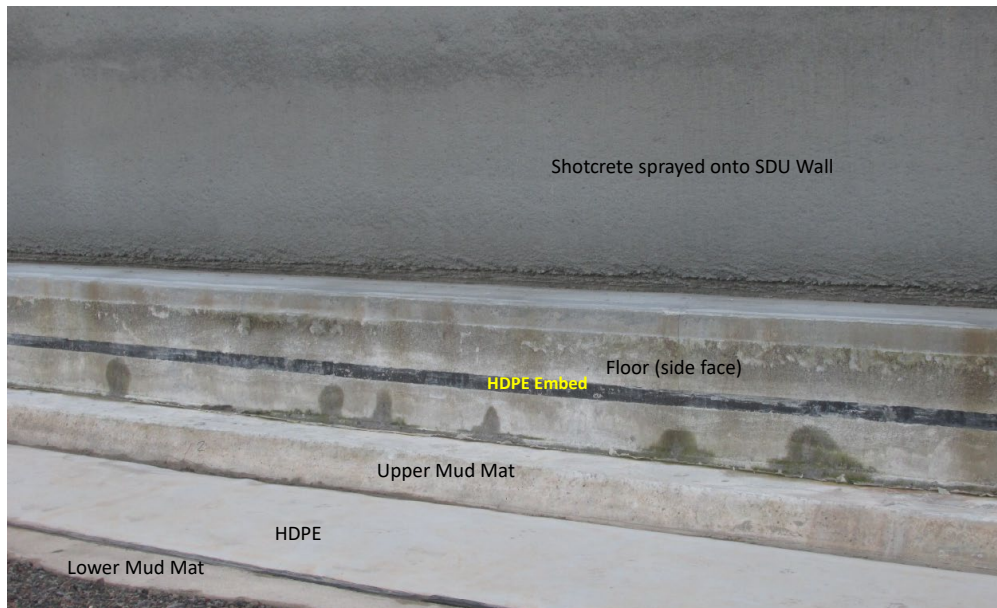
Figure 2.3-5: Observed Leak from First Leak Tightness Test of SDU 6, November 2015 (5 of 6)
