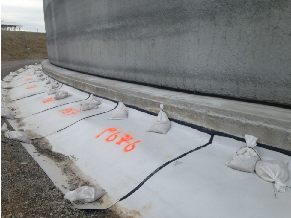
Figure 2.3-8: Installation of HDPE Over the Mud Mats
