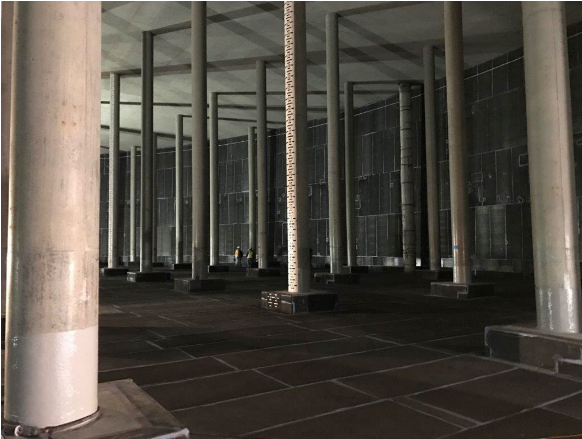
Figure 2.3-7: Interior of SDU 6 After Liner Installation (Fall 2016)
