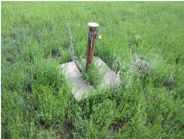
Photo #7 Typical view of some of the on-site groundwater monitoring wells on the site.
