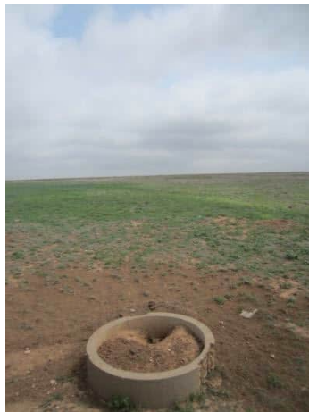
Photo #39 View of a sewer access conduit of the sewage pipeline in the pastureland east of the Pantex Village.
