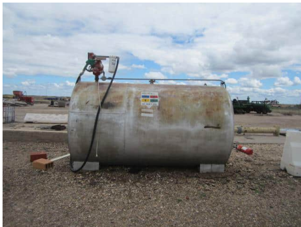
Photo #81 View of the diesel AST north of the former building 2-4.
