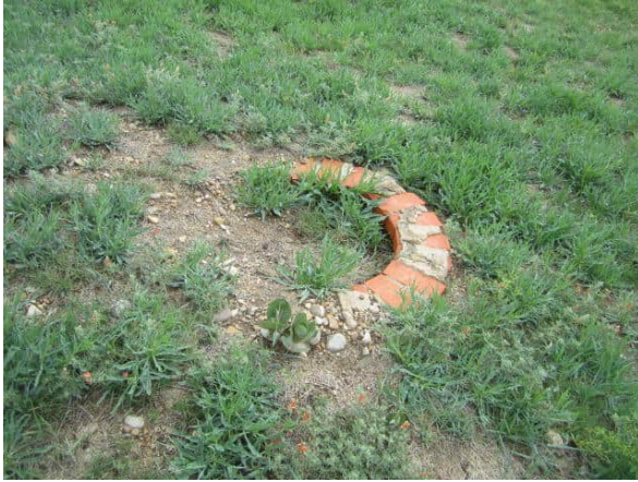
Photo #31 View of a filled in sewer manhole on the former residential area.
