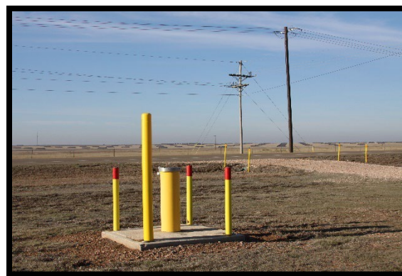
Fig. 3.20. In-situ bioremediation system well near Zone 11.
