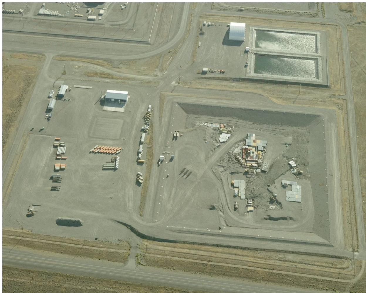
Figure 2-3. View of ICDF Landfill and Evaporation Ponds looking east (photo taken September 11, 2009).
