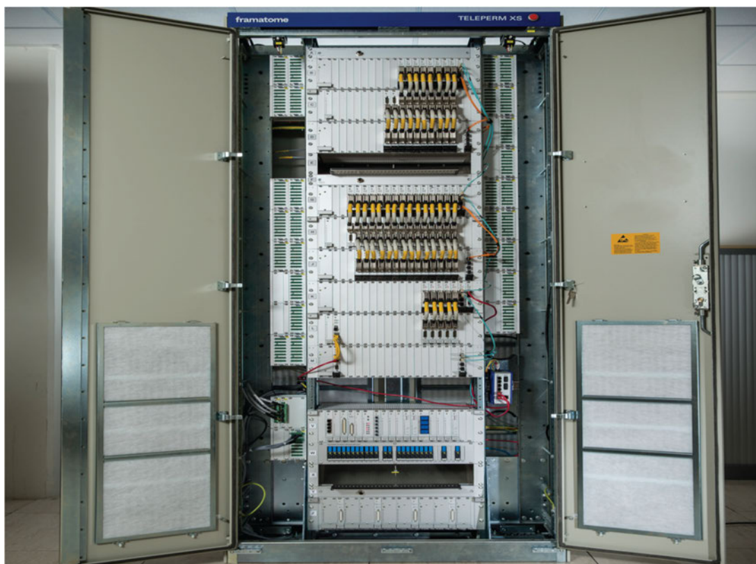
Figure 1: TELEPERM XS Compact in Cabinet 3
