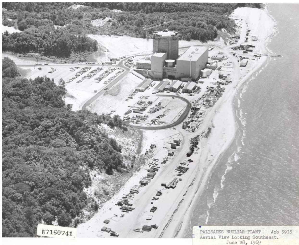
Figure I-16 A Photograph from June 28, 1969, Looking Southeast over the Palisades Nuclear Plant Site. Note the Cleared Vegetation and Road Cut into the Sand Dune to the Left of the Reactor Vessel Building and the Land Grading and Vegetation Clearing along the Beach to the South of the Site. This Location Is Where Both Cooling Towers Exist Today. Source: HDI 2024-TN10670.
