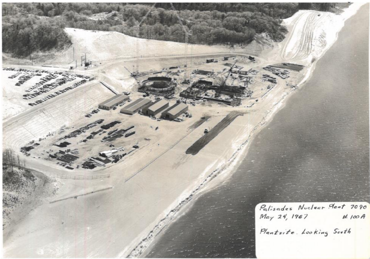
Figure I-10 A Photograph from April 25, 1967, Looking Southeast over Palisades Nuclear Plant Site. Note the Cleared Vegetation and Road Cut into the Sand Dune to the Left of the Circular Footprint of the Future Reactor Vessel Building and the Land Grading and Vegetation Clearing along the Beach to the South of the Site. Source: HDI 2024-TN10670.
