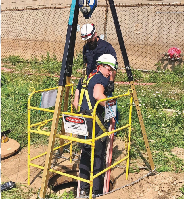
Inspector Shawn Lichvar descends into an underground vault at the Beaver Valley nuclear power plant, securely harnessed, to inspect safety-related electrical cables at the western Pennsylvania facility.
