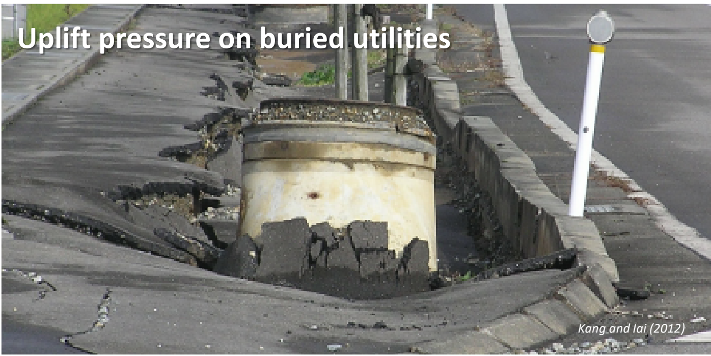
Bearing capacity failure, settlement
