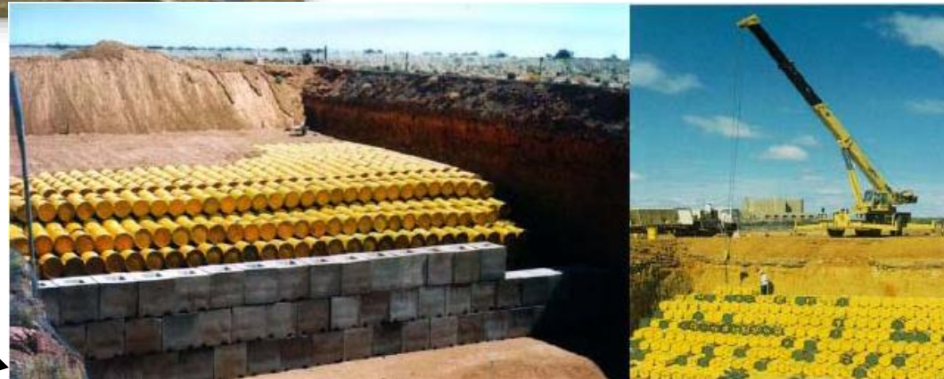
Vaalputs waste repository -Experimental Trench A1 (buried concrete drums) 1986
