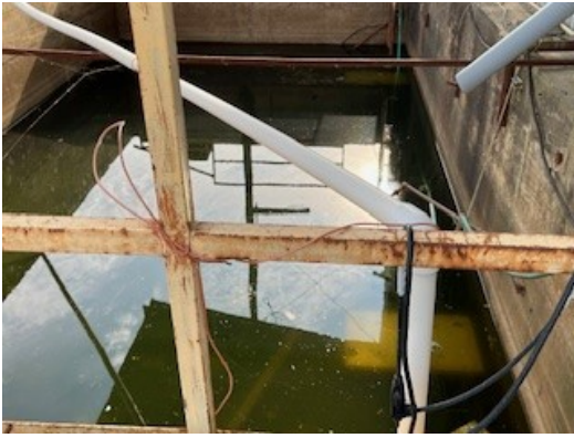
Pond 3 Area (pond, nearby monitoring stations and sumps)
