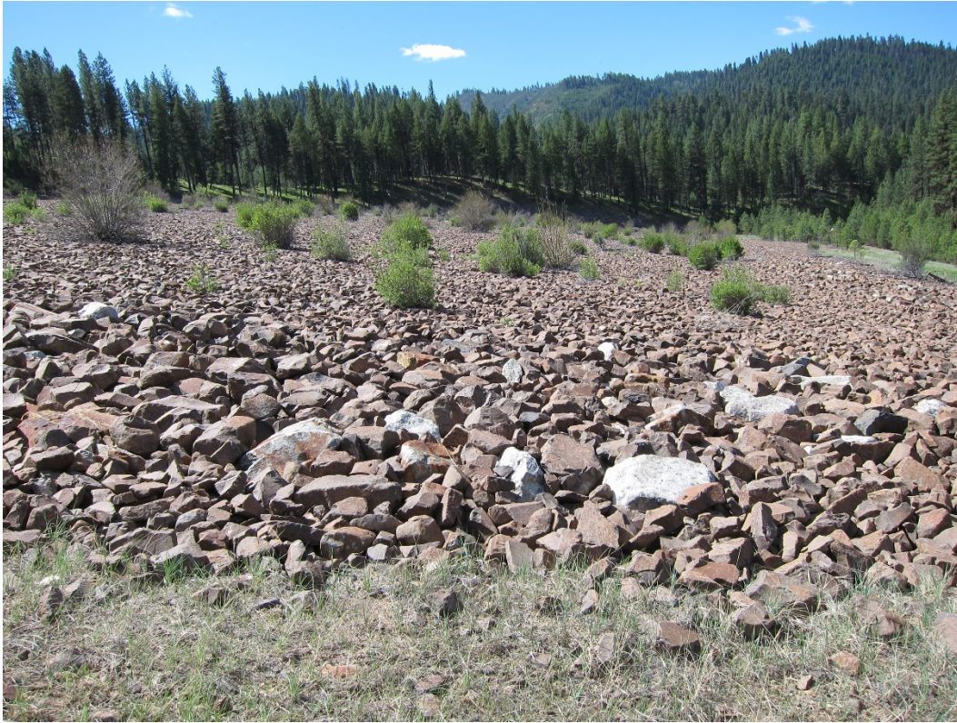
Figure 3: Disposal cell with apron riprap in foreground (looking north to south)
