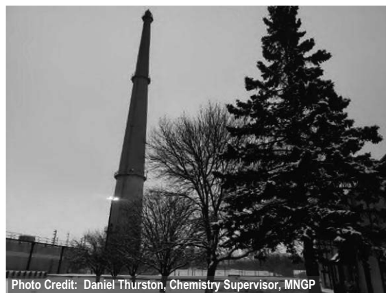
Plant Stack, used for dispersing treated gaseous effluents, Monticello Nuclear Generating Plant in Winter
