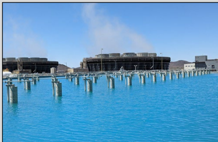
Palo Verde Nuclear Generating Station spray pond
