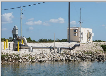
Well used to adjust salinity in the Turkey Point Nuclear Generating Station's cooling canals
