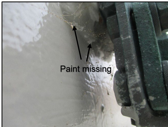
16. 270° ground strap underside
