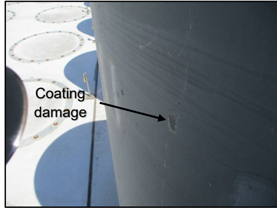
89a. Coating damage overpack SW quadrant (close-up)
