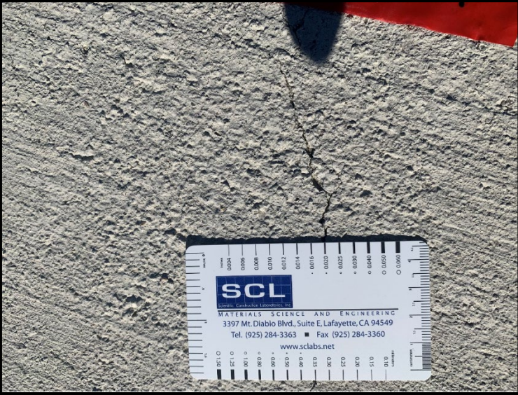
3. Closeup of cracking on Pad 5 near joint
