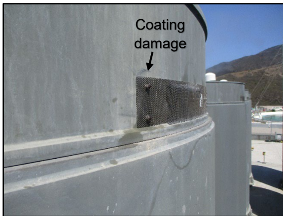
31. Upper east vent coating damage from nut removal
