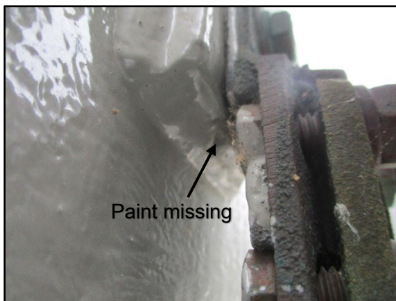
18. 90° ground strap underside
