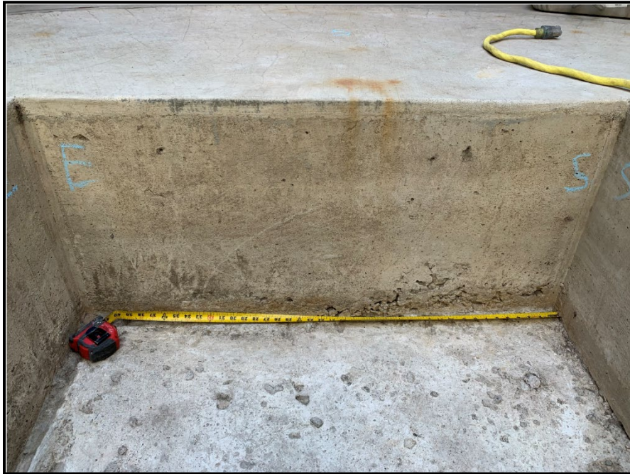
7. Area of poor consolidation in sump of the CTF structure
