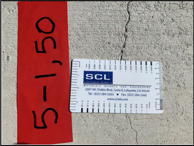
3. Closeup of cracking on Pad 5 near joint
