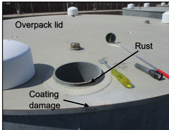
20. NE lid-stud pipe chipped paint and rust, chip at lid edge
