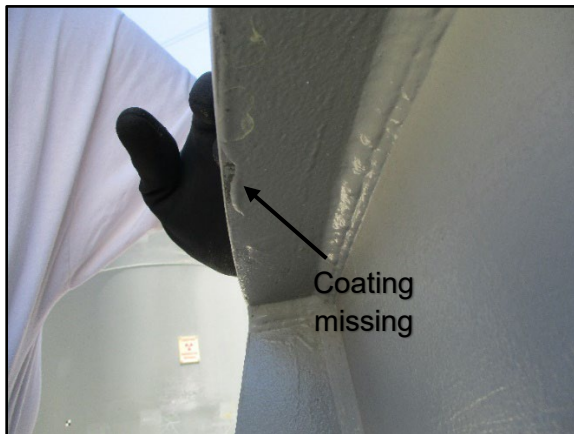
58. Missing outer coating between anchor studs #10 & #7
