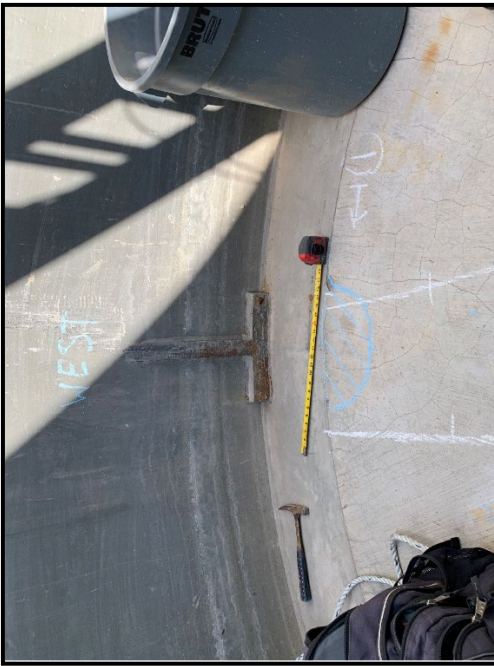
6. Delamination on west side of the CTF structure
