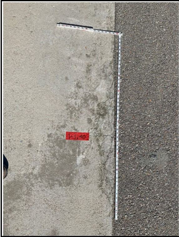
1. Delaminated concrete on Pad 1 eastern side
