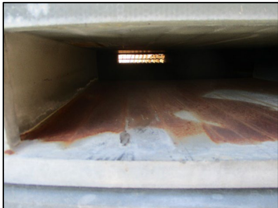
7. West upper overpack vent (gamma shield out) rust
