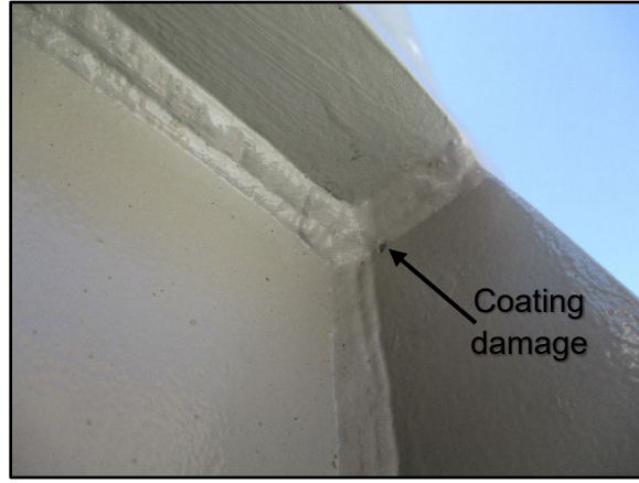
72. Chipped outer coating at anchor stud #1
