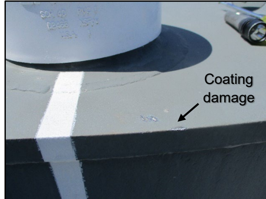
86. Coating damage at edge NE quadrant
