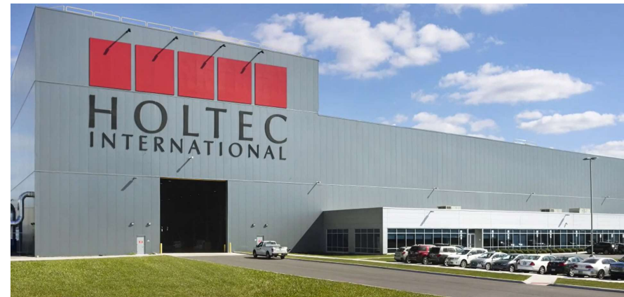
Holtec's Advanced Manufacturing Division (AMD) Designed and Constructed for Fabrication of SMR-300
