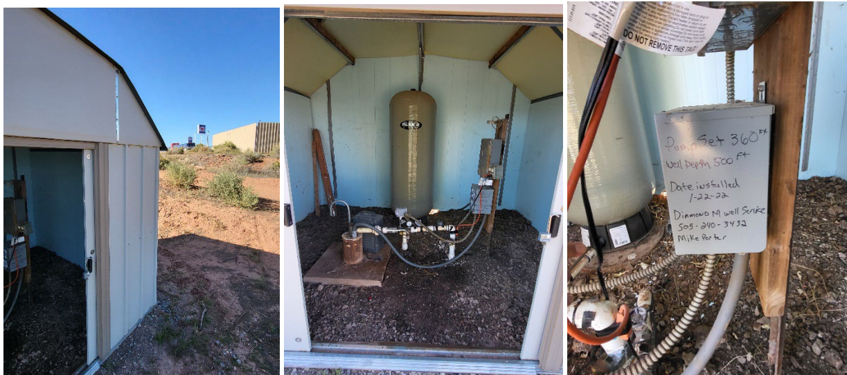
Photographs 9a, 9b, 9c – BSAG-26 sample location. Private supply well.
