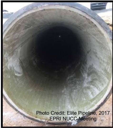
CIPP: Cured-in- Place-Pipe
