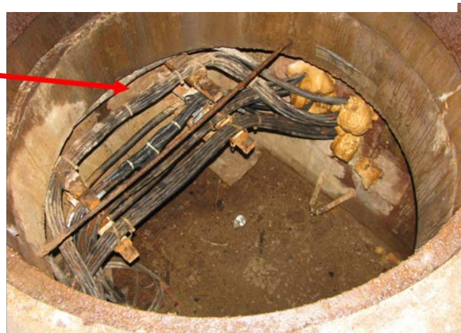
Manhole with Spliced Cables
