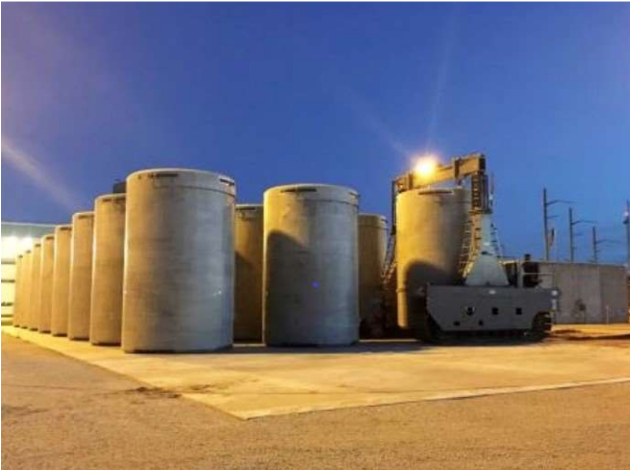
Spent Fuel Dry Cask Storage
