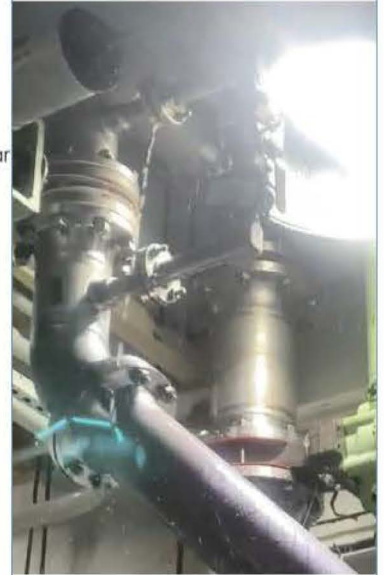
You're the inspector, find the leaking flange above.
