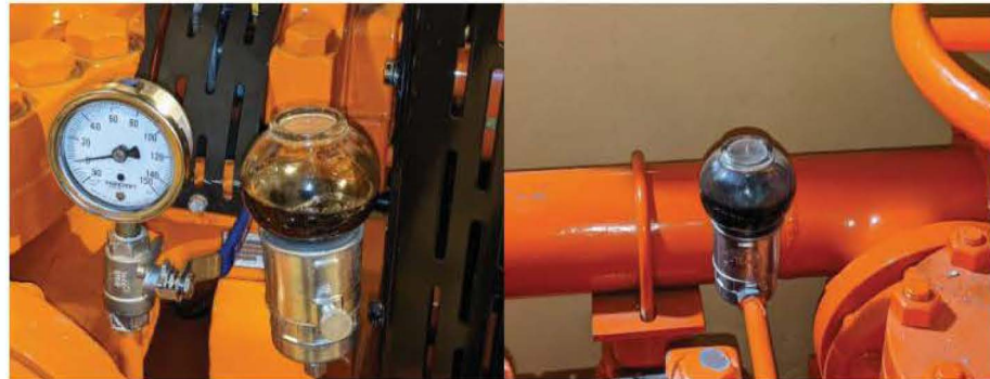
FLEX AFW Pump #1 Oil Bubbler
