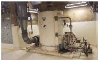
'B' Hydrogen Recombiner Installed in Unit 1 auxiliary building (Note the wall-mounted placard on the left side of the photo, shown enlarged later).
