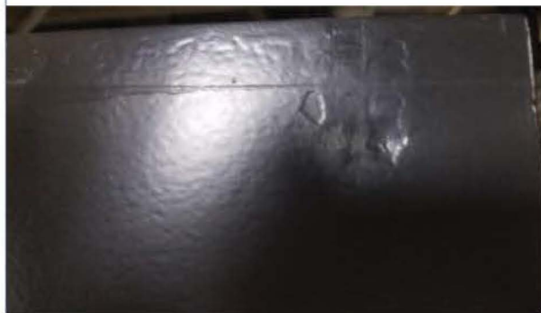
Fire door showing minor damage caused over time by door coordinator arm striking the door without a rubber roller.
