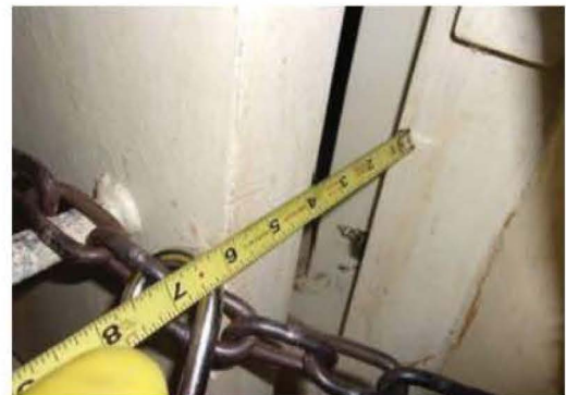
Gap in the locked doors leading to the RX head stand area.
