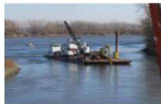
Barge Conducting Dredging of Discharge Canal at Cooper
