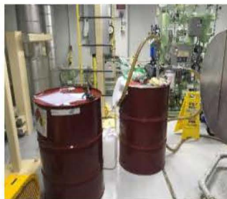
Unattended drums of lube oil in EDG enclosure without a fire prevention permit.
