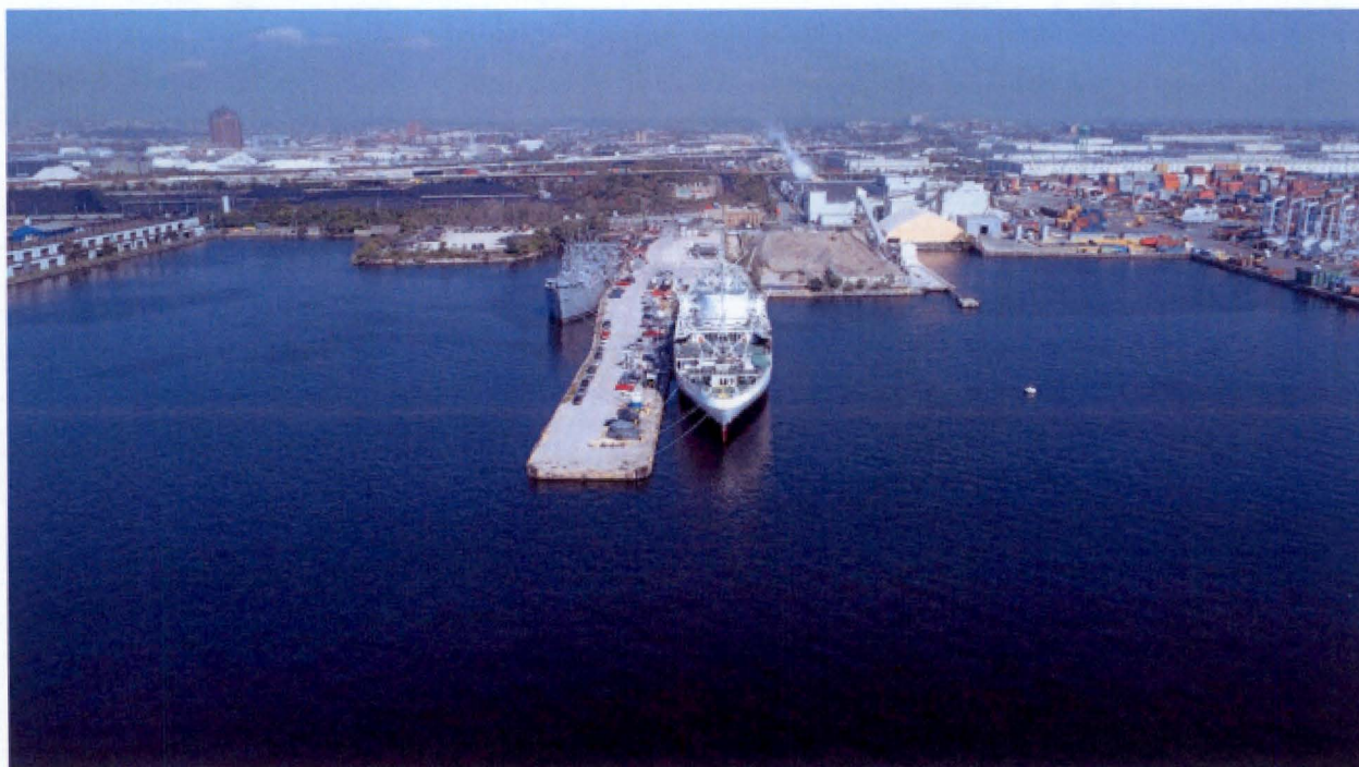
Figure 1-10 NSS at Pier 13, September 2023, looking northward
