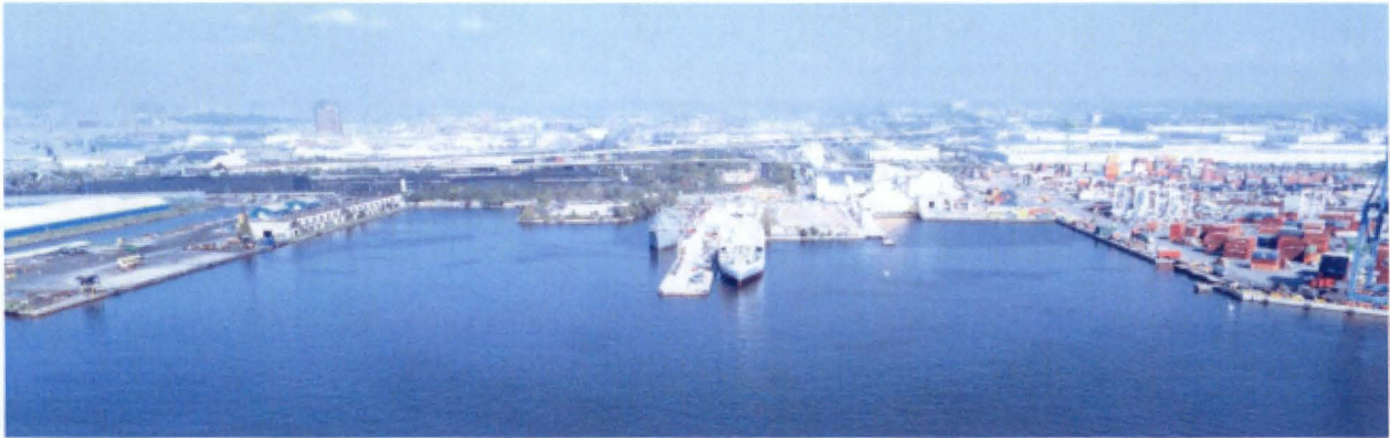
Figure 1-11 NSS at Pier 13, September 2023, looking northward
