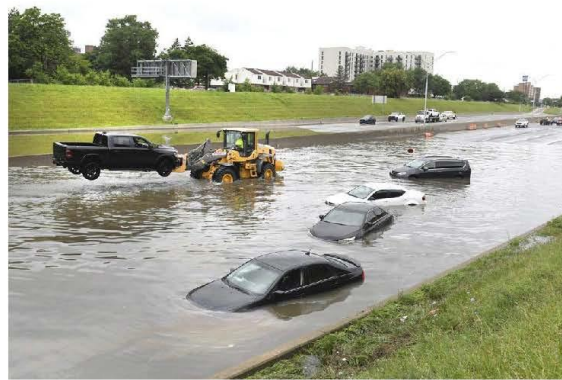
Interstate 75 in Detroit, on 26, 2021. A Detroit-area water service provider denied flooding claims based on an independent review that found the flooding was due to the amount of rainfall and not a defect in its collection system. ( Max Ortiz/Detroit News via AP File )
