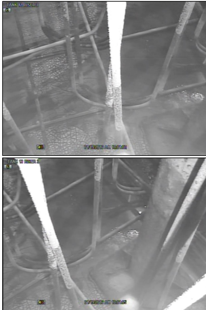
Figure 1. Residual WIR on the Floor of the Tank 12H Primary Appears Similar to Mud Cracks. Light Reflects off a Pool of Water beyond the Column in the Bottom Image. Date of Video: January 19, 2016.
