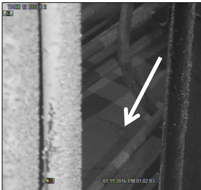
Figure 3. Photo of Bleed-Water Segregation Occurring in Grout Poured into the Tank 12H Primary. The Dark Outline Surrounding a Freshly Deposited Lobe of Grout is Segregated Water Separating from the Grout Mass. Date of Video: January 19, 2016.
