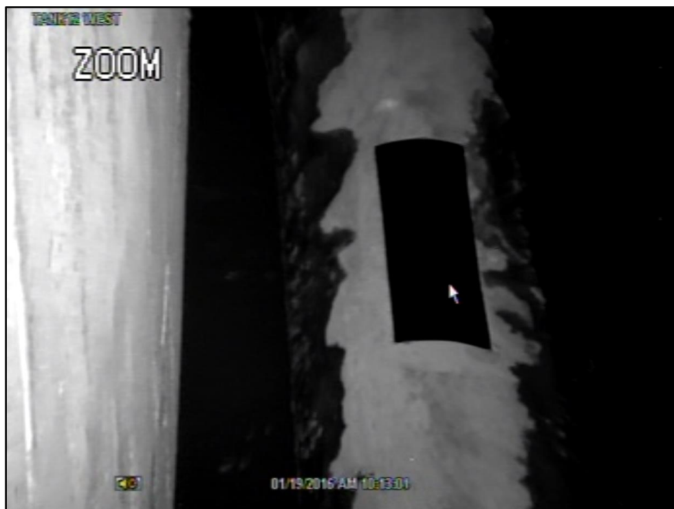
Figure 5. Photograph of Rectangular Ventilation Register in the Annulus, as viewed from the West Riser. Date of Video: January 19, 2016.
