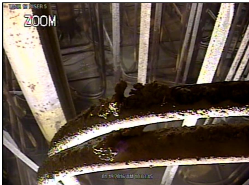
Figure 2. Residual WIR on cooling coils within the Tank 12H Primary. Date of Video: January 19, 2016.
