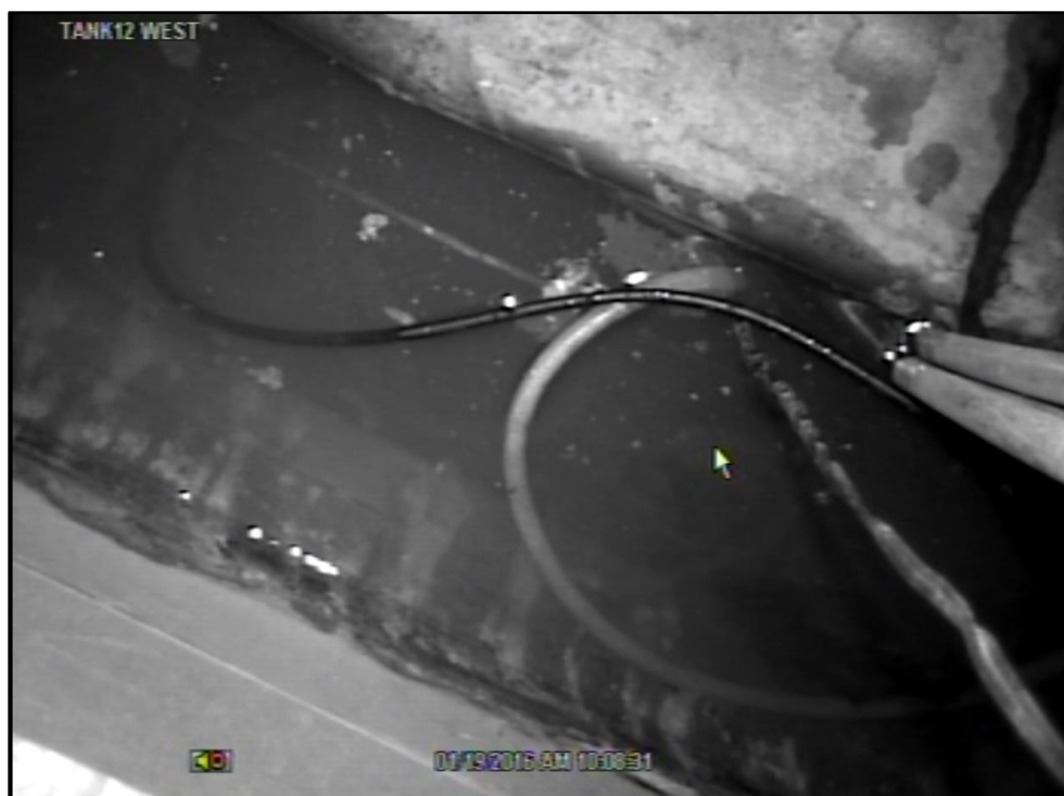
Figure 4. Groundwater In-Leakage in the Annulus, as viewed from the West Riser. Date of Video: January 19, 2016.
