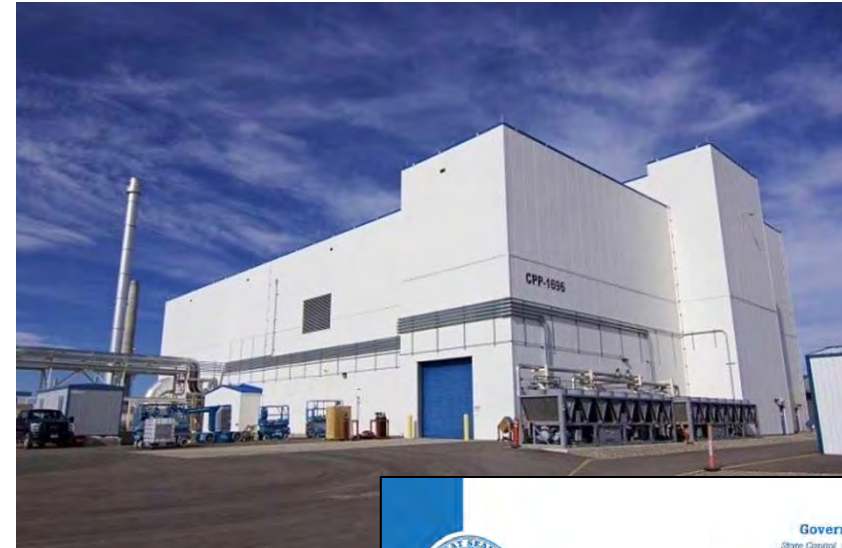
Integrated Waste Treatment Unit at INL
