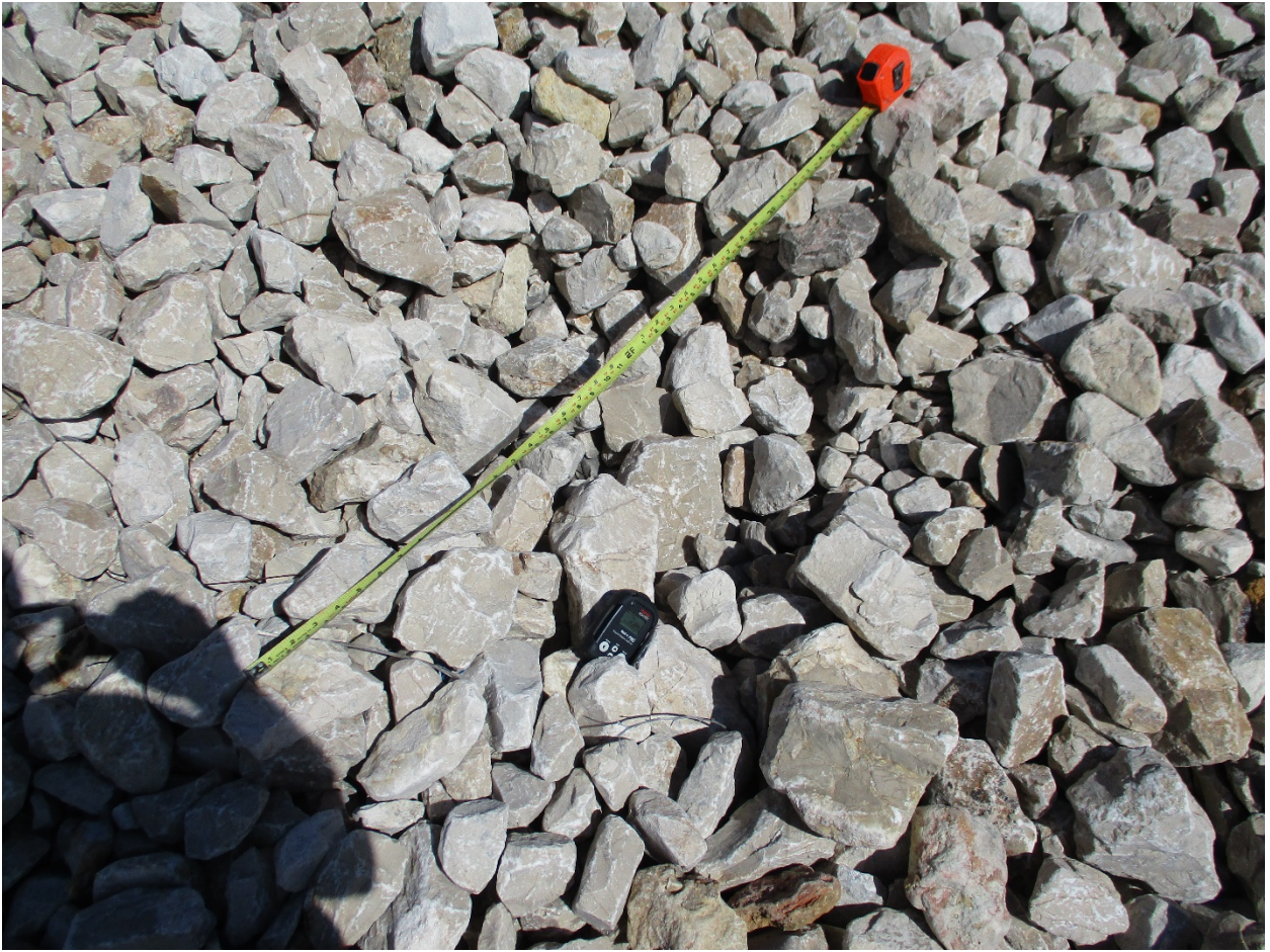
Figure 5: South embankment rip-rap minor settlement
