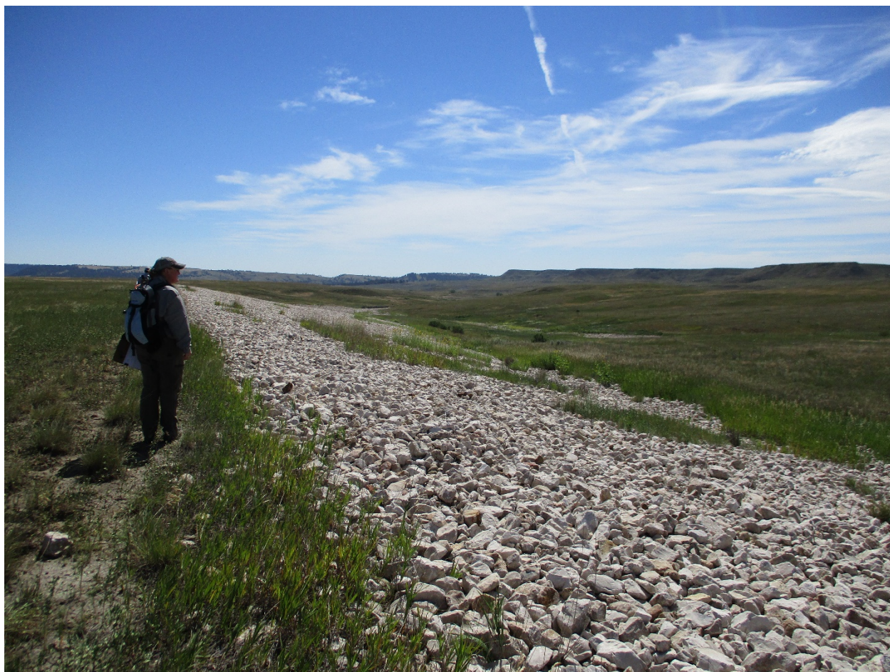
Figure 2: Tailings embankment with rip-rap cover, southeast corner (looking west)
