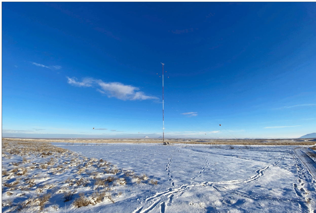
Figure 2.7-53: CFPP Tower, November 2022, View to the East-Southeast
