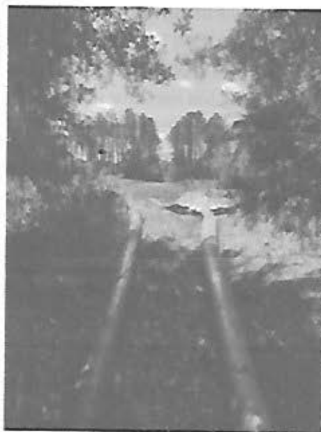
Figure 2: Construction site drainage in Flagler County, photo by Stephanie Hezel
