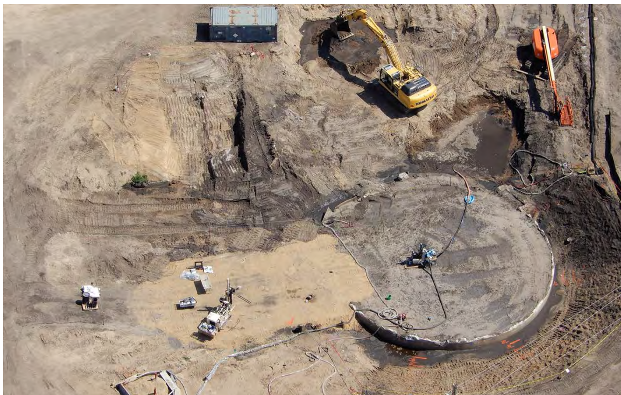
Figure 10. Survey Unit L1-SUB-TDS B (RPGA Sump) at time of GeoProbe Sampling from June 26, 2019, to July 12, 2019
