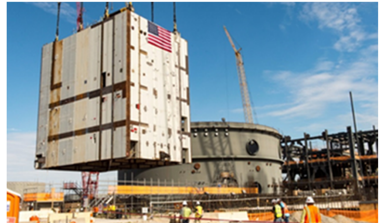
AP1000® Use of Steel Modules
