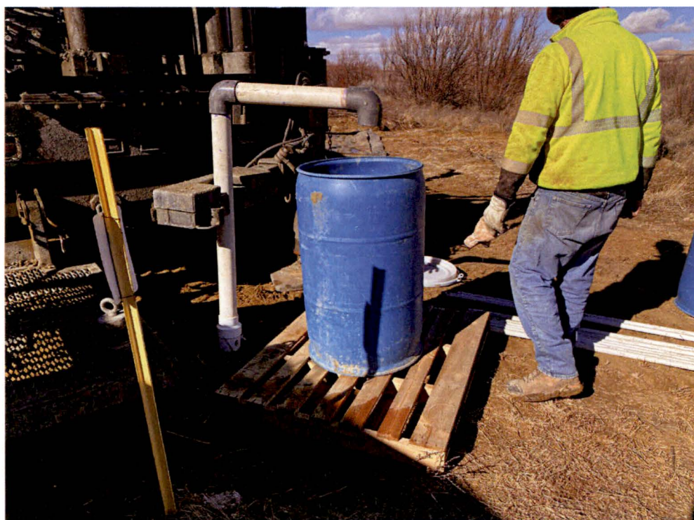
Photograph 4 -Yellow Jacket staff air-lifting sediments from 5-04 ALL during P&A
