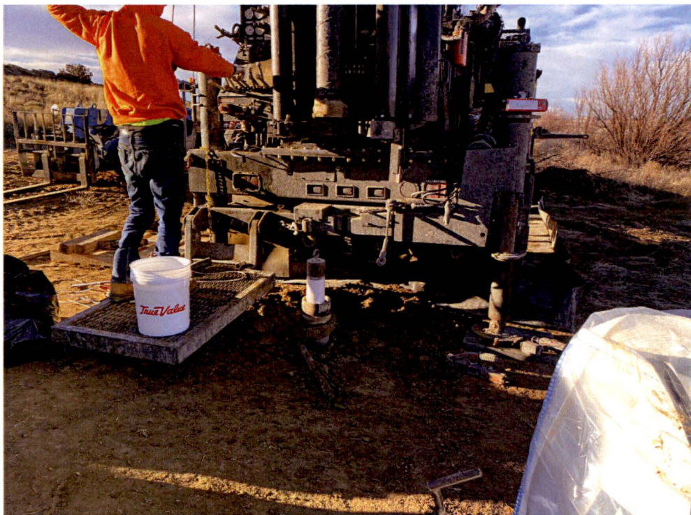
Photograph 2 -Yellow Jacket staff during well completion at 5-04 ALL-R
