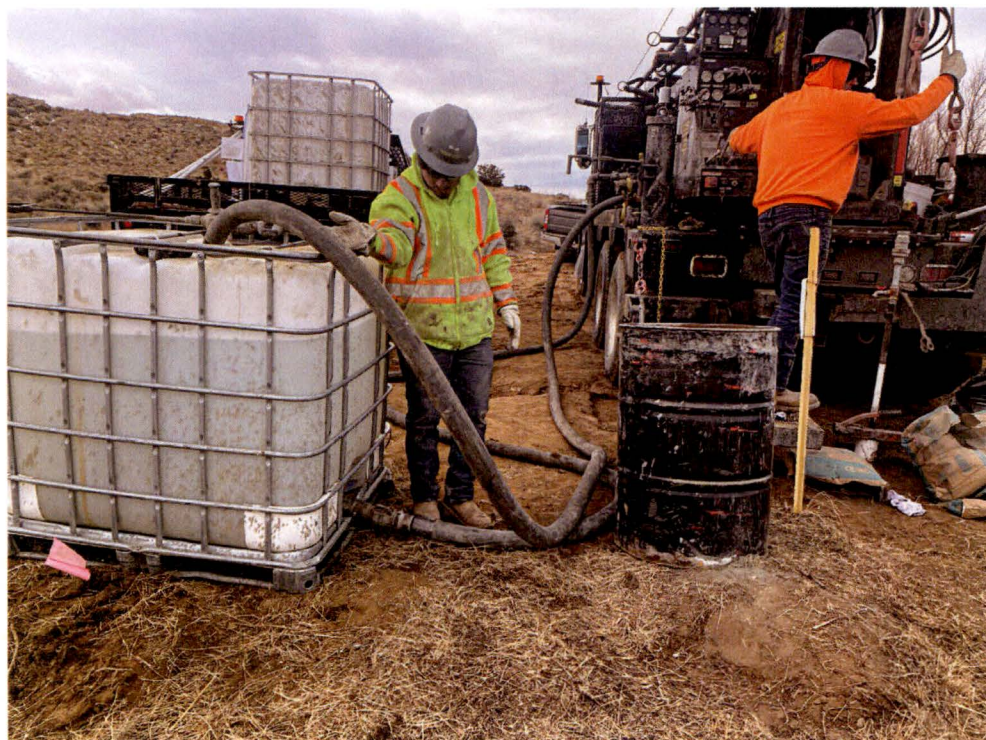
Photograph 6 -Yellow Jacket staff mixing grout for 5-04 ALL P&A
