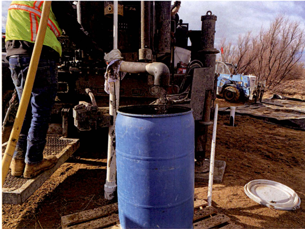
Photograph 5 -Yellow Jacket staff air-lifting sediments from 5-04 ALL during P&A
