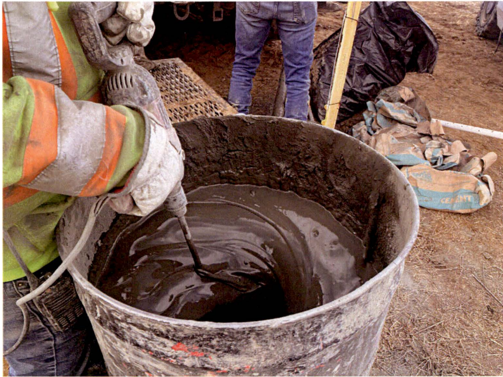
Photograph 7 -Yellow Jacket staff mixing grout for 5-04 ALL P&A
