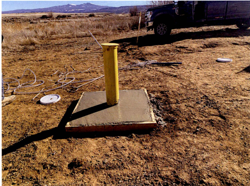
Photograph 8 -Finished 5-04 ALL-R surface completion (foreground) with marker for 5-04 ALL (background)
