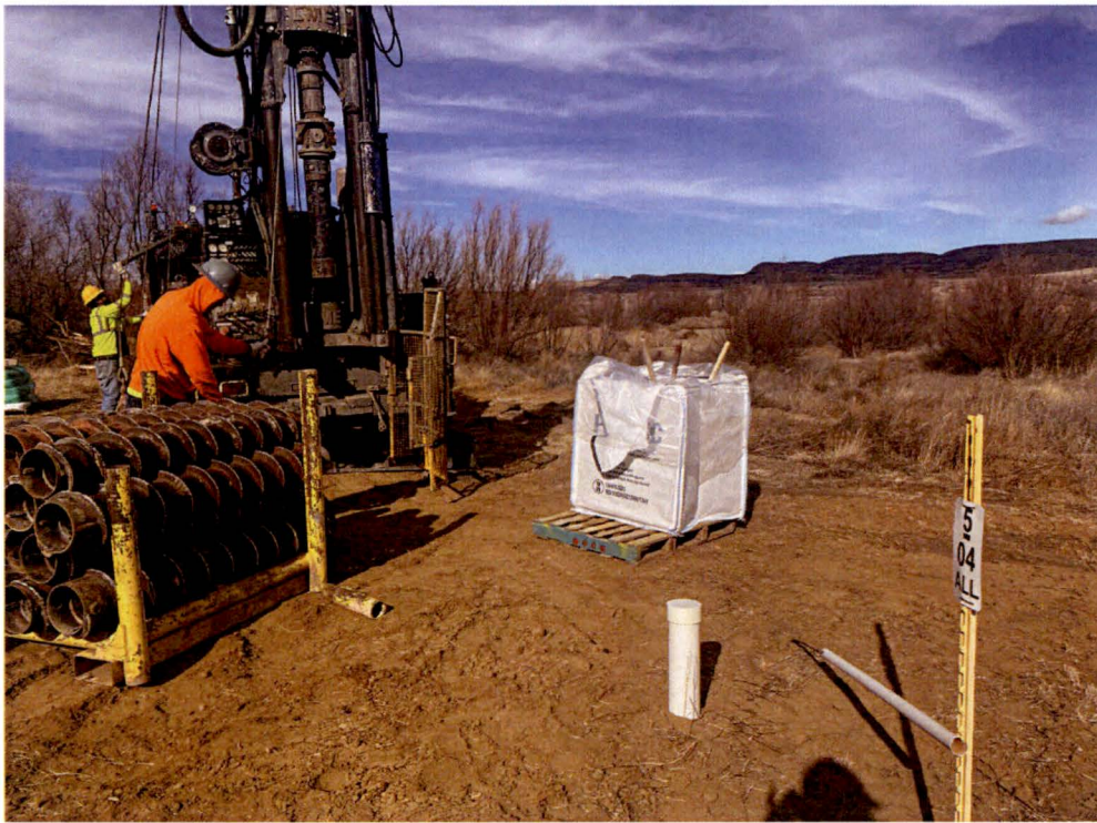
Photograph 1 -Yellow Jacket staging supplies and equipment for replacement well
