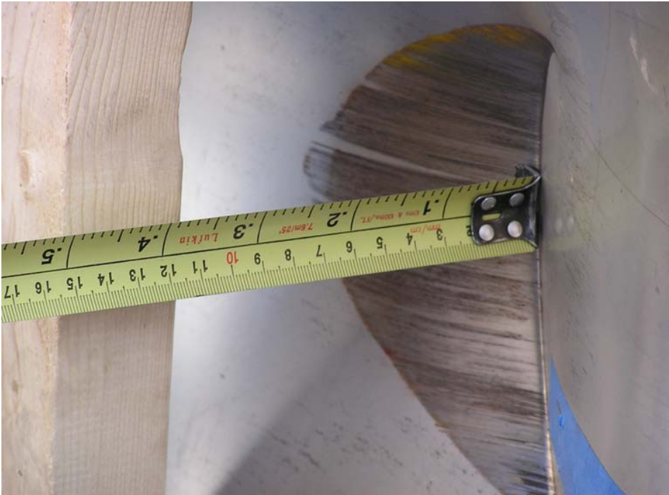
Figure 2-32 Close Up of Puncture Damage
