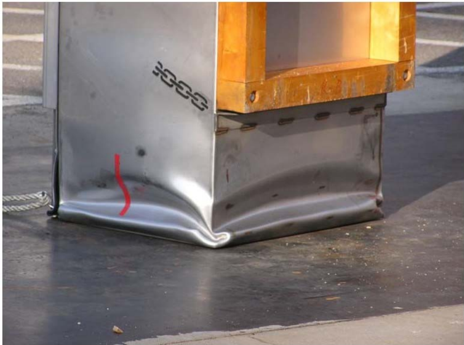
Figure 2-34 Damage from End Impact (Bottom and Side)
