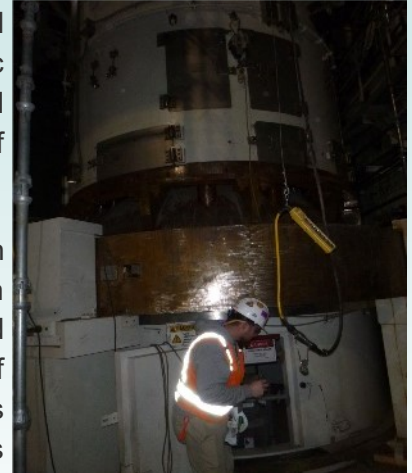
Resident Inspector Brian Griman performing containment closeout inspection prior to Integrated Leak Rate Test
