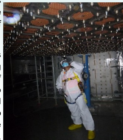
Senior Construction Inspector Raju Patel inspecting reactor internals after hot functional testing
