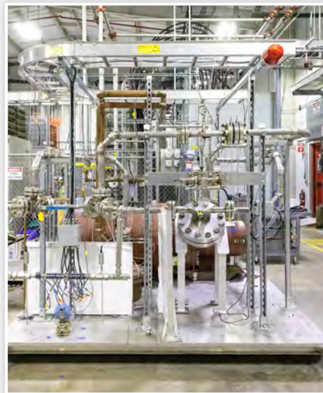
Helium flow loop test stand. Helium provides advantages over water-based cooling
