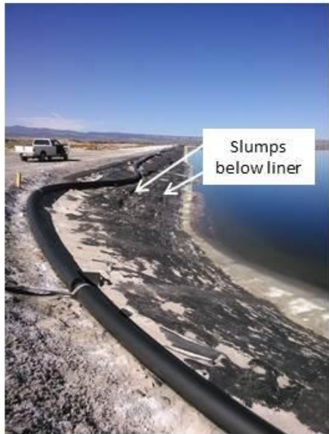
Figure 1 – Slumps below liner at east end of south inslope, EP1
