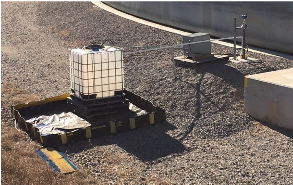
Figure 2.3-8: East Sump After Construction
