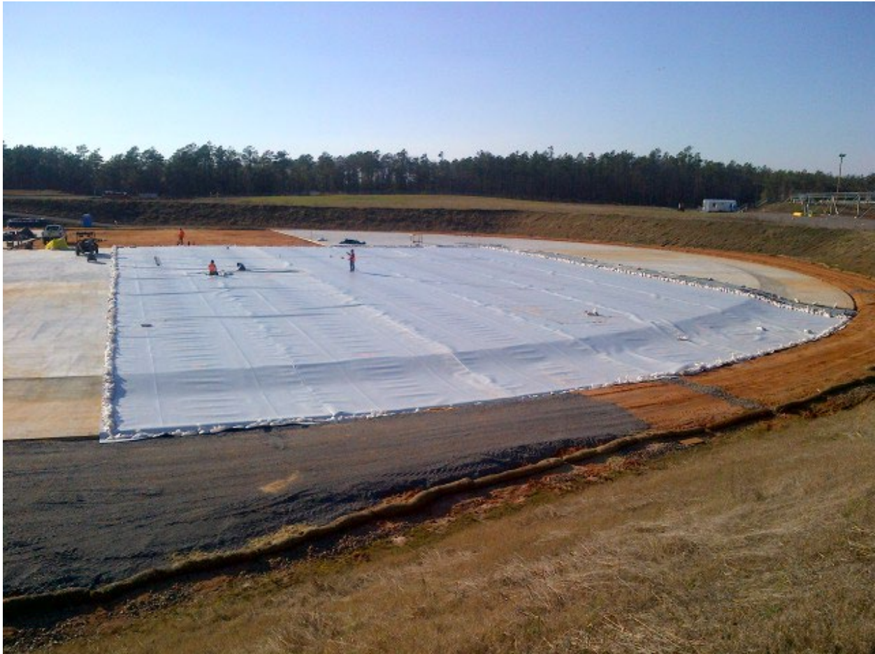
Figure 2.3-3: Installation of HDPE above the Lower Mud Mat of SDU 6
