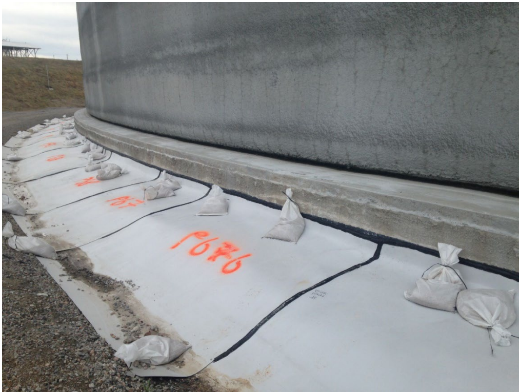
Figure 2.3-6: Installation of HDPE Over the Mud Mats
