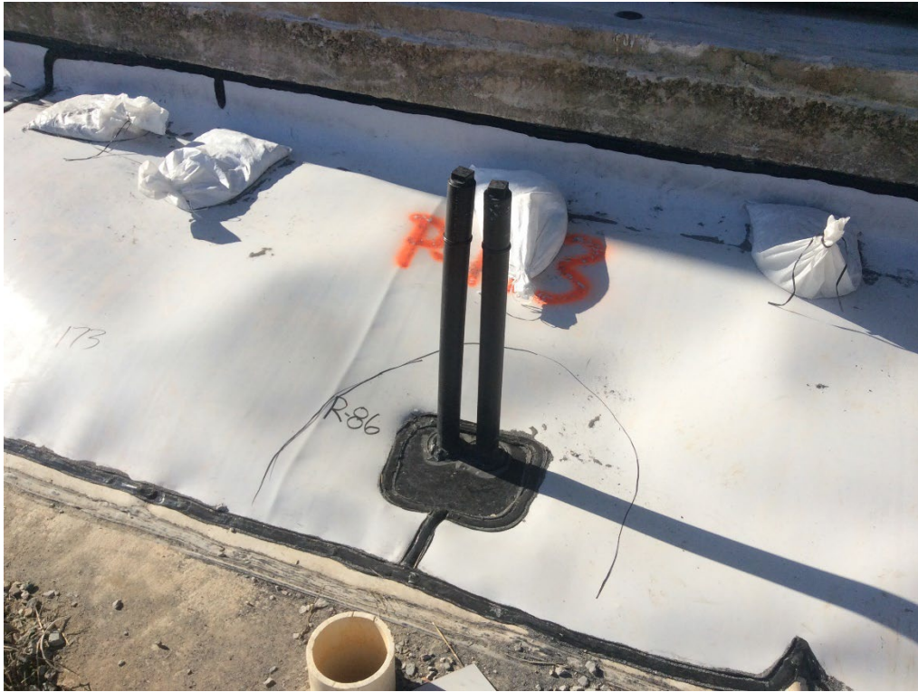
Figure 2.3-7: Installation of HDPE Over the Mud Mats at East Sump
