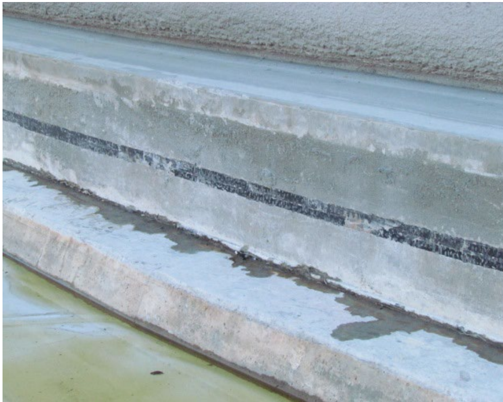
Figure 2.3-5: Edge of SDU 6 Floor Showing the HDPE Embed (Photo Taken During 1 st Leak Tightness Test)
