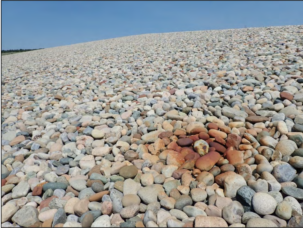
PL-5. Lightning Strike on Side Slope
