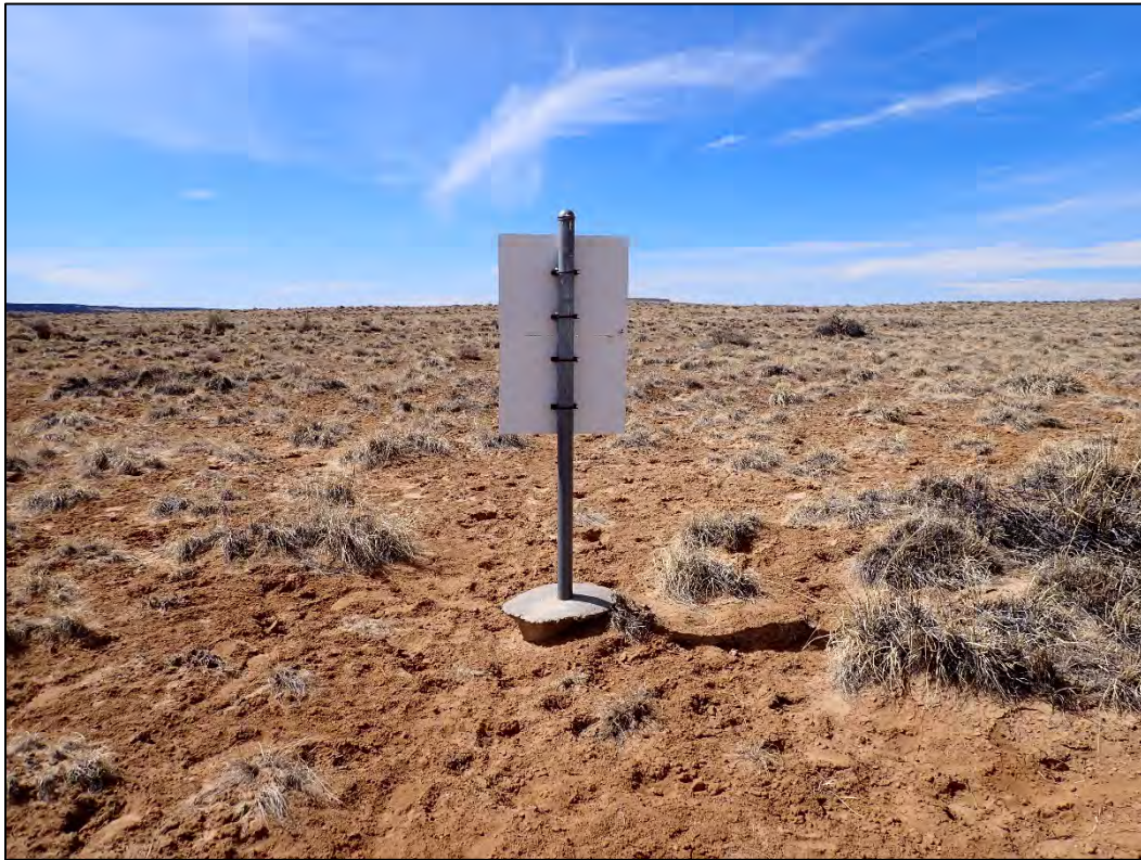
PL-3. Erosion Around Base of Perimeter Sign P12 (Stable)
