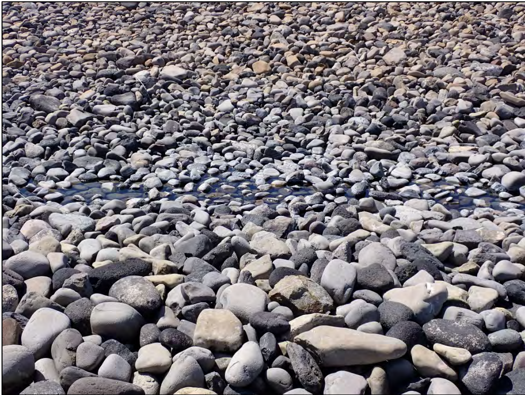
PL-8. Standing Water in Southeast Cell Toe Drainage
