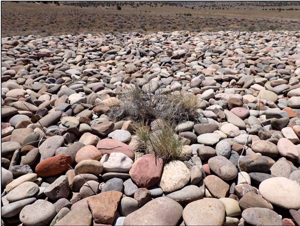
PL-7. Vegetation Growing on Disposal Cell Cover
