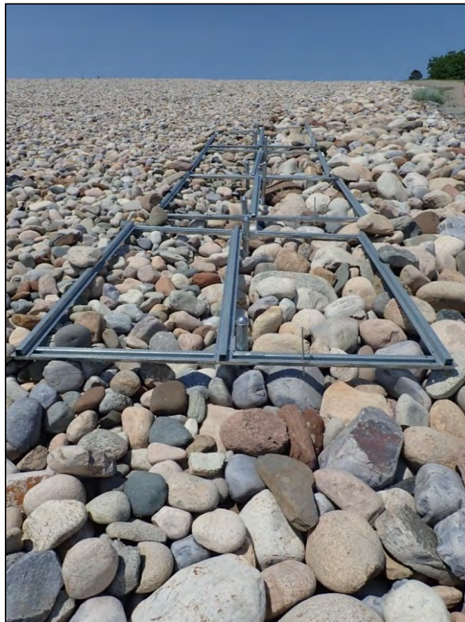
PL-4. Monitoring Grid over Linear Depression
