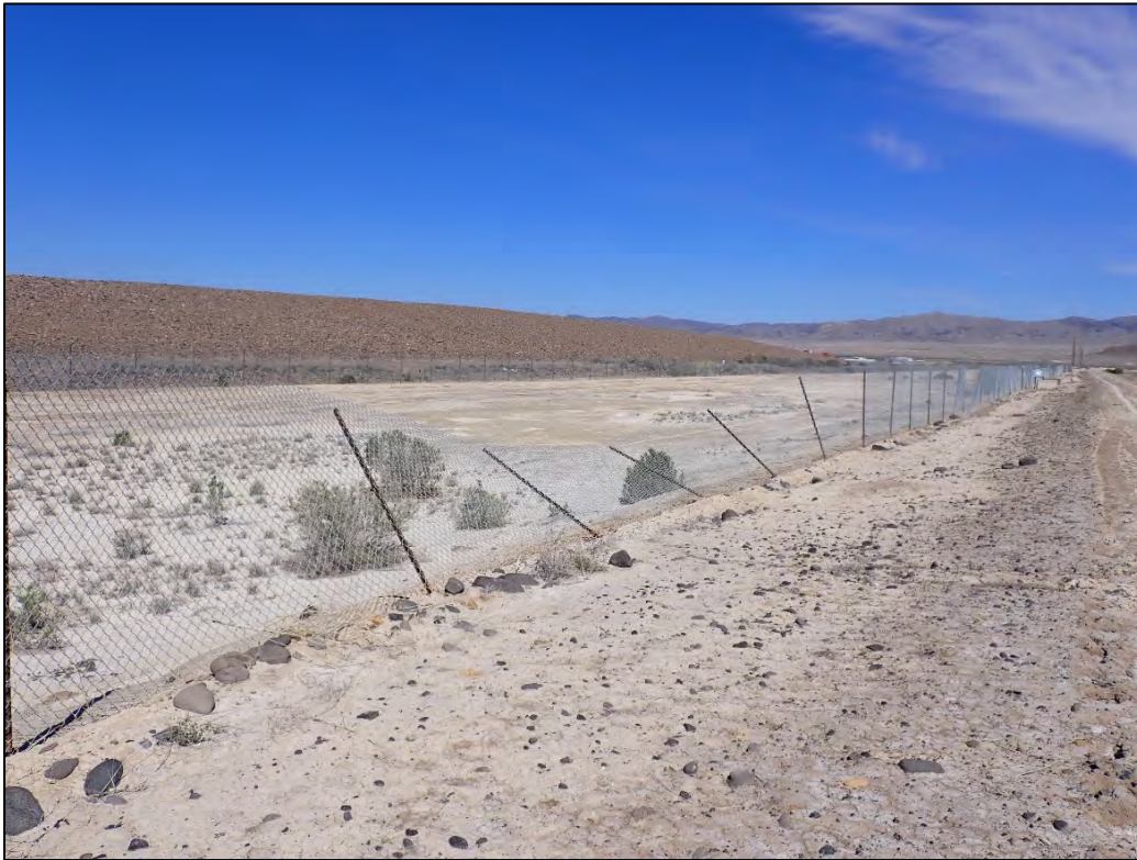
PL-1. Down Fence Along South Side of Cell
