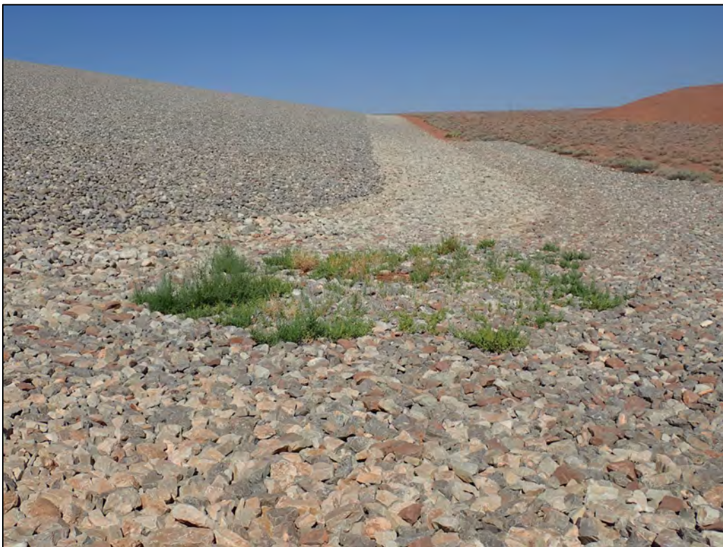
PL-16. Northeast Toe Drain
