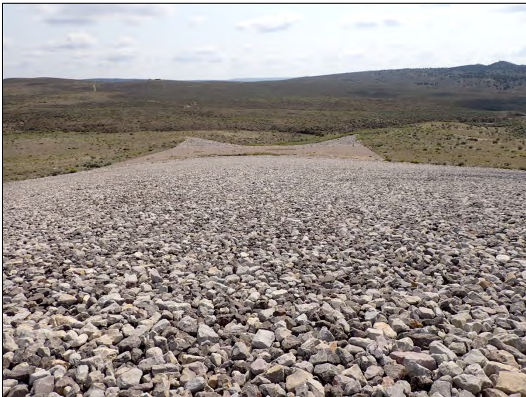
PL-10. Disposal Cell Eastern Side Slope and Cobble Blanket
