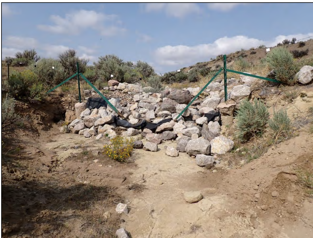
PL-12. Exposed Geofabric in Diversion Channel No. 1 Outlet
