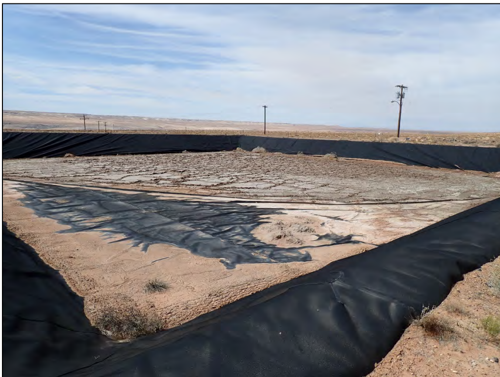
PL-12. Evaporites and Windblown Sand in Inactive Evaporation Pond
