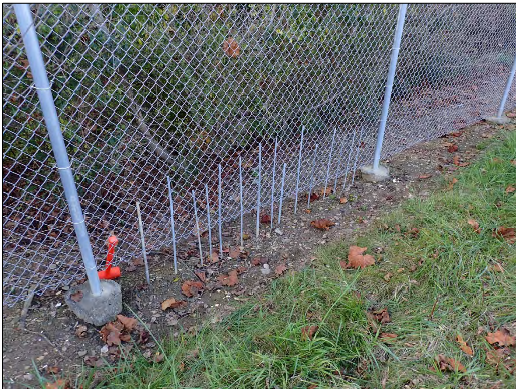
PL-4. New Slats in Fence at Erosion Area
