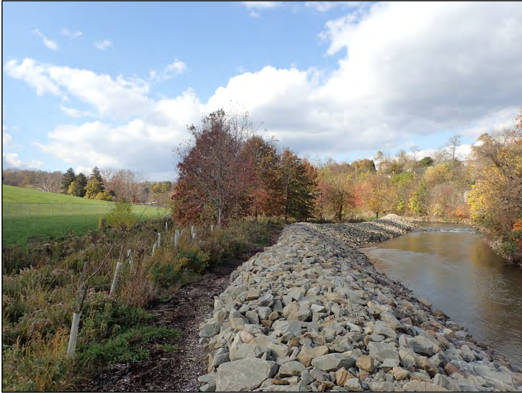
PL-11. Riparian Area and Riprap-Armored Streambank
