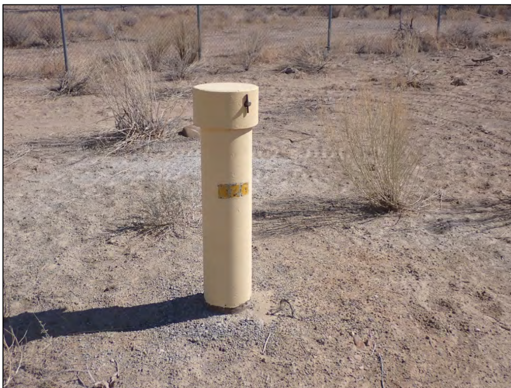
PL-7. Faded Identification Numbers on Monitoring Well 0176
