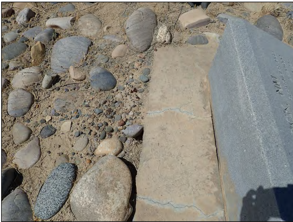
PL-2. Cracks and Erosion in Concrete Base of Site Marker SMK-1
