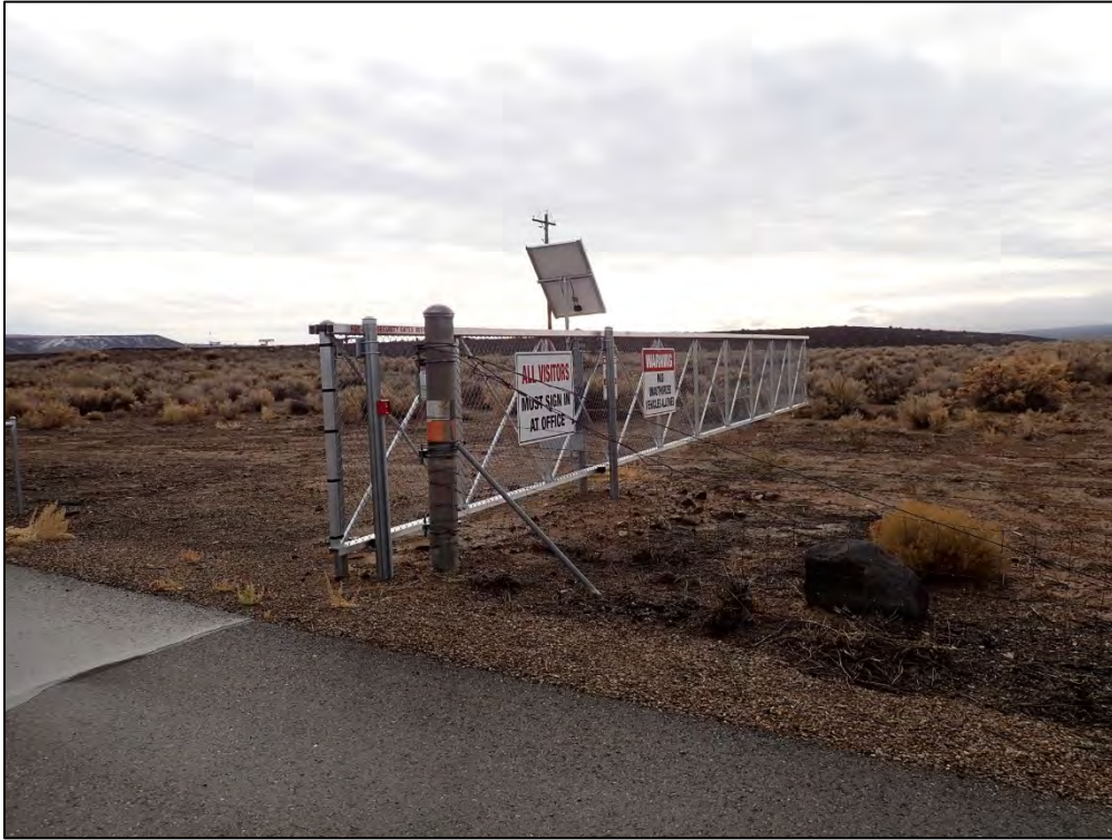
PL-1. Solar-Powered Site Entrance Gate
