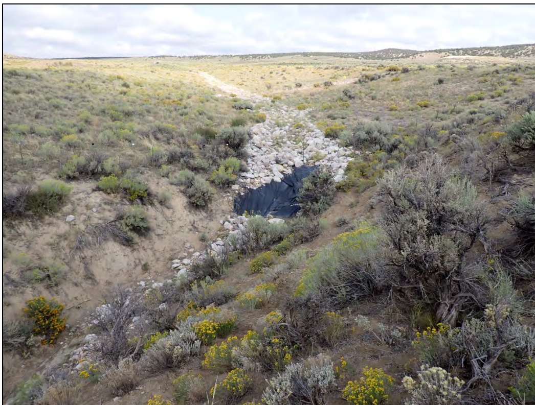
PL-13. Exposed Geofabric in Swale No. 1 Outlet
