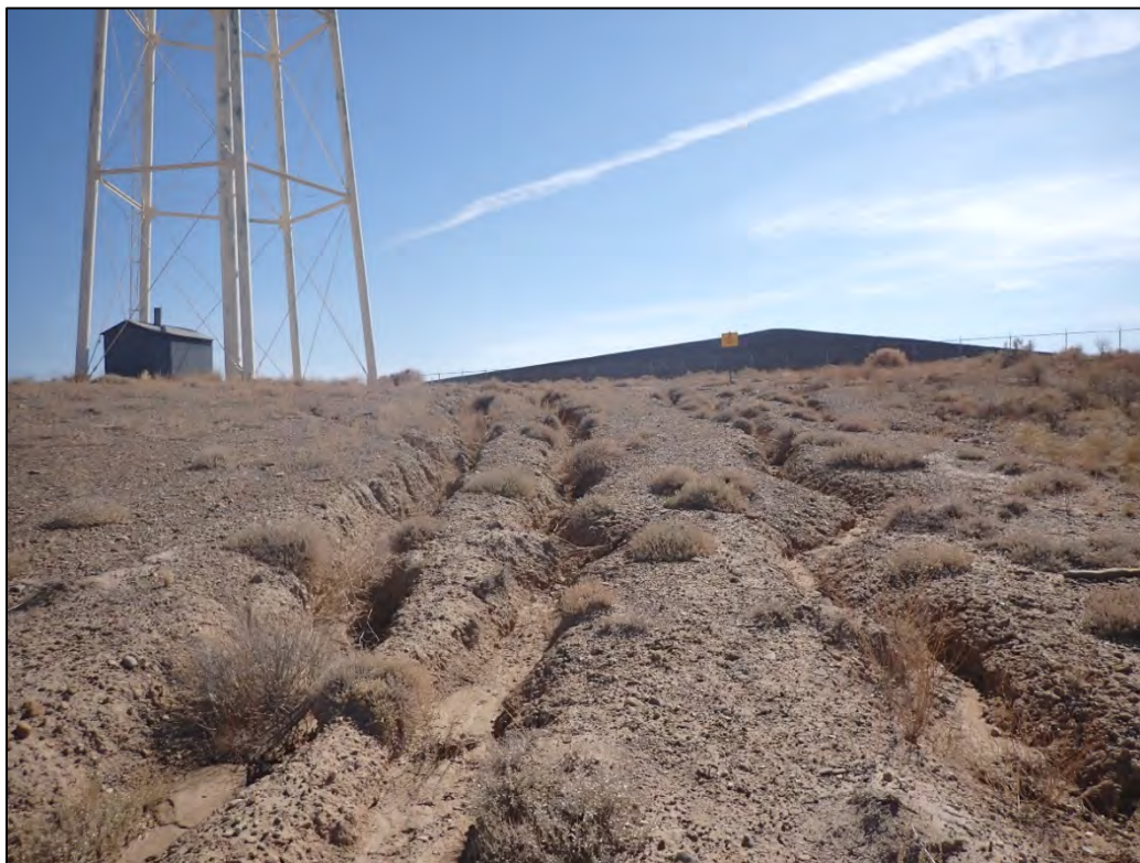
PL-15. Soil Erosion (Offsite)
