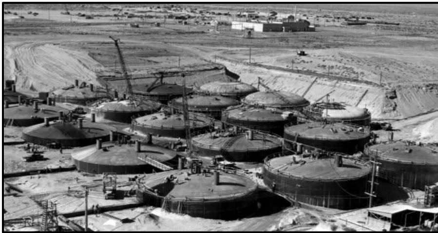
Figure 2-1 Tank Farm Under Construction
