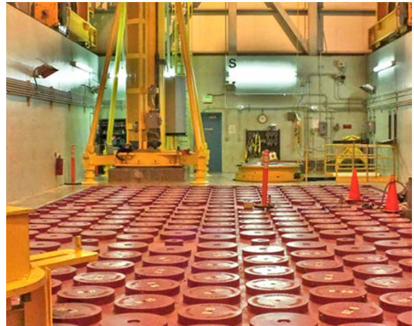
Figure 4. Inside the Fort St. Vrain Independent Spent Fuel Storage Installation (CH2M-WG Idaho, LLC 2012).
