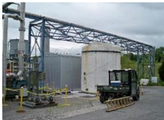
Figure 3.20. The Chromium Water Treatment System
