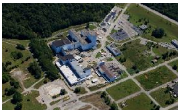
Figure 3.14. K-1200 Complex before decontamination and demolition
