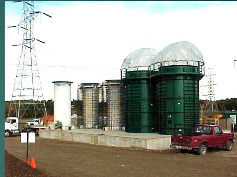
Dry Spent Fuel Casks on Concrete Pad at Nuclear Power Plant Site
