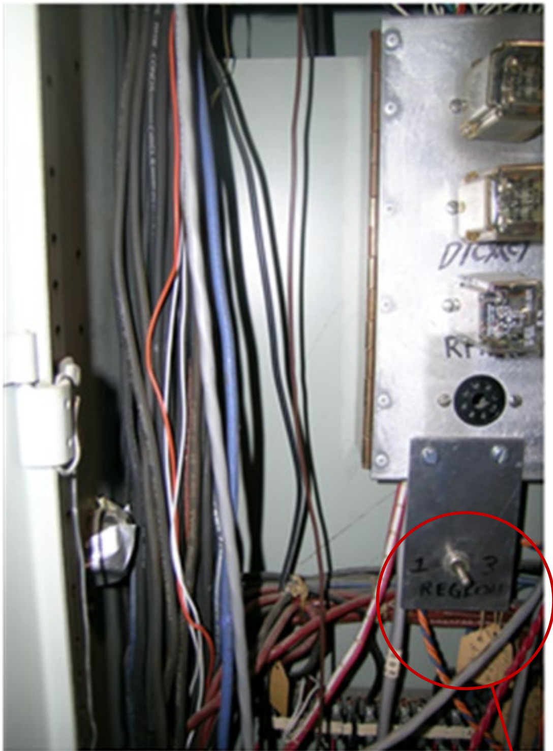
Figure 4-6 – Previous Core Dolly Override Switch
