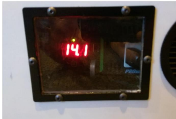
Figure 3 Battery voltage LED display
